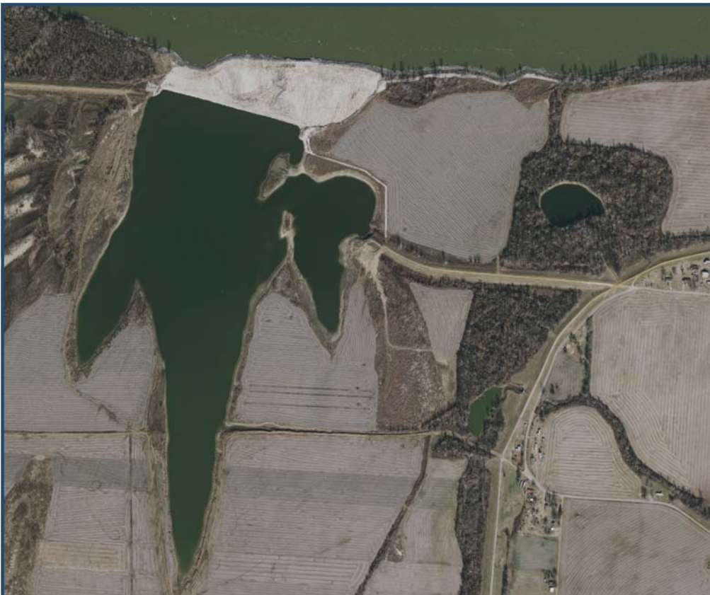
A view of the riprap cap placed over the dredge fill material placed once the bank had been reestablished.
