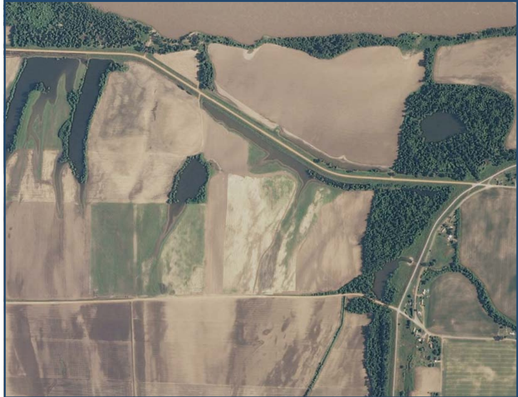
View of the Sheep Ridge Road Spur Levee at Merriwhether-Cherokee in October 2010, prior to the attempted natural river cutoff.
