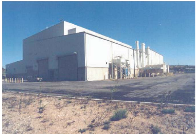
Building 1900 (Integrated Refurbishment Facility)
