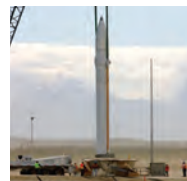
GBI Placement into Silo
