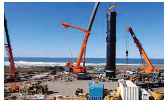
Emplacement of Silo
