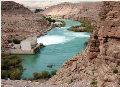
KAJAKI DAM The dam was built with U.S. funds in the 1950s, and the U.S. Agency for International Development installed two turbines in the 1970s to provide electrical power as far away as Kandahar City. After 2001, there was a plan to install a third turbine but it did not occur. The area was the scene of heavy fighting in 2007, and over the years Coalition personnel and contractors had difficulty getting to the site because of Taliban attacks, with travel largely limited to military convoy or helicopters.
