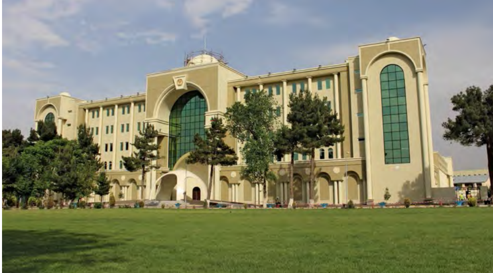
New MoD Headquarters in Kabul. (AFCEC photo)
