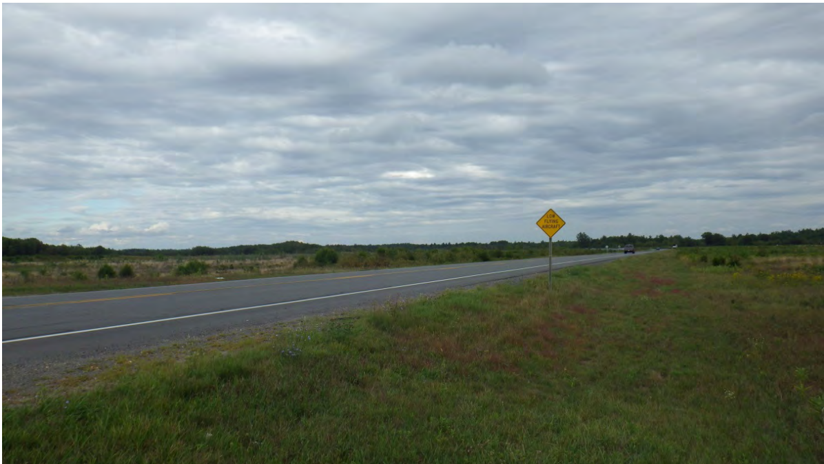
Photo Description: Just south of Highway 3A toward northeast (helicopter training area). Representative of current public view.
