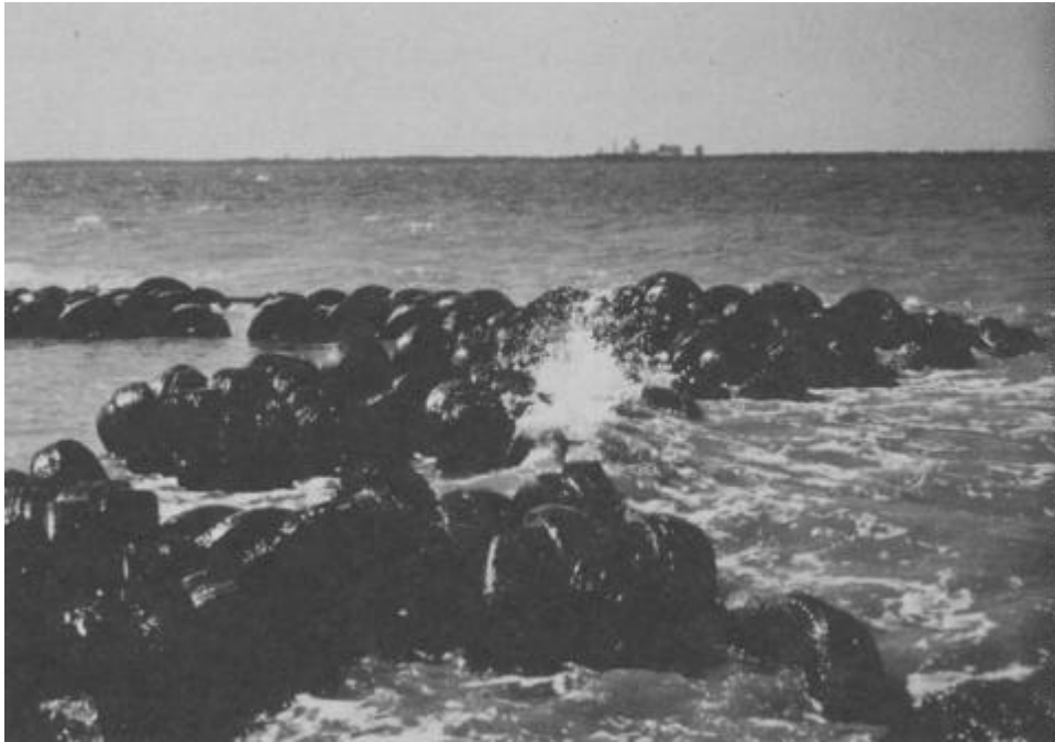
Figure 5-2. A floating tire breakwater installed at Gaillard Island, Alabama, to protect newly planted marsh from moderate wave energies
