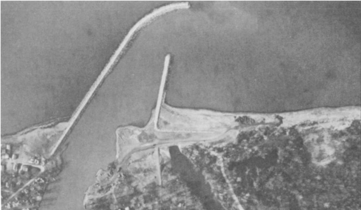
Figure A-38. Aerial photograph of Cattaraugus Creek mouth after improvements.
