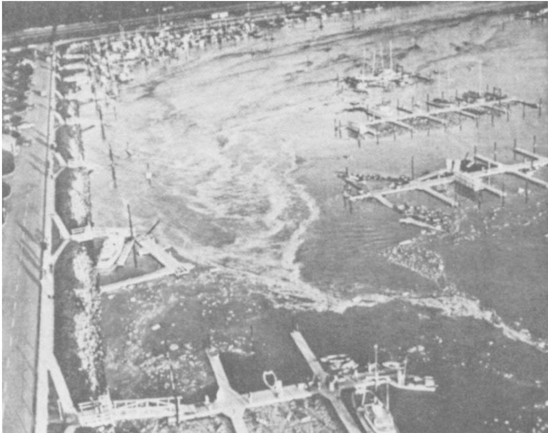
Figure 3-2. River flood damage at Ventura Marina, California.
