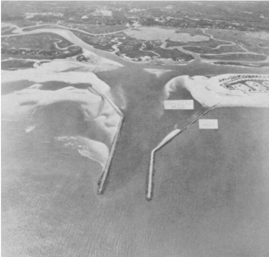
Figure A-47. View of Murrells Inlet project, as constructed in 1981.
