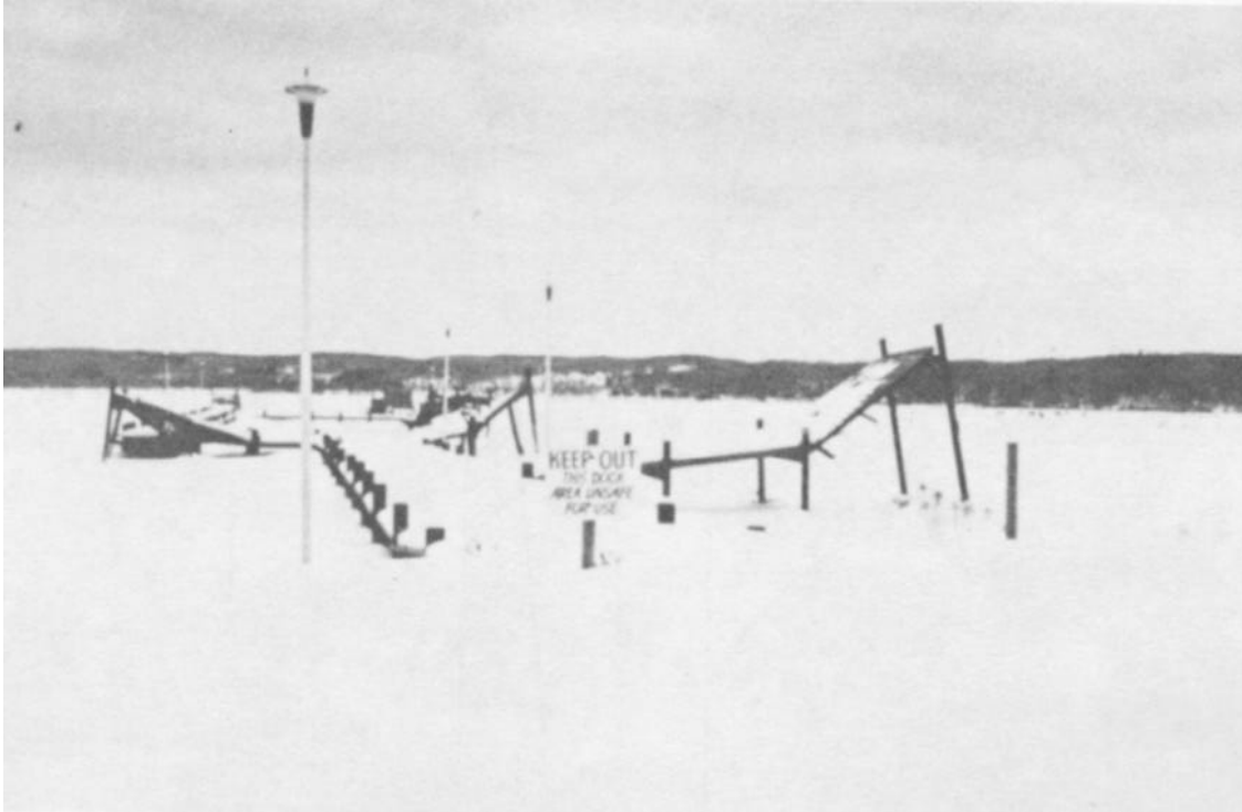
Figure 3-13. Damage to piles caused by the vertical movement of ice.
