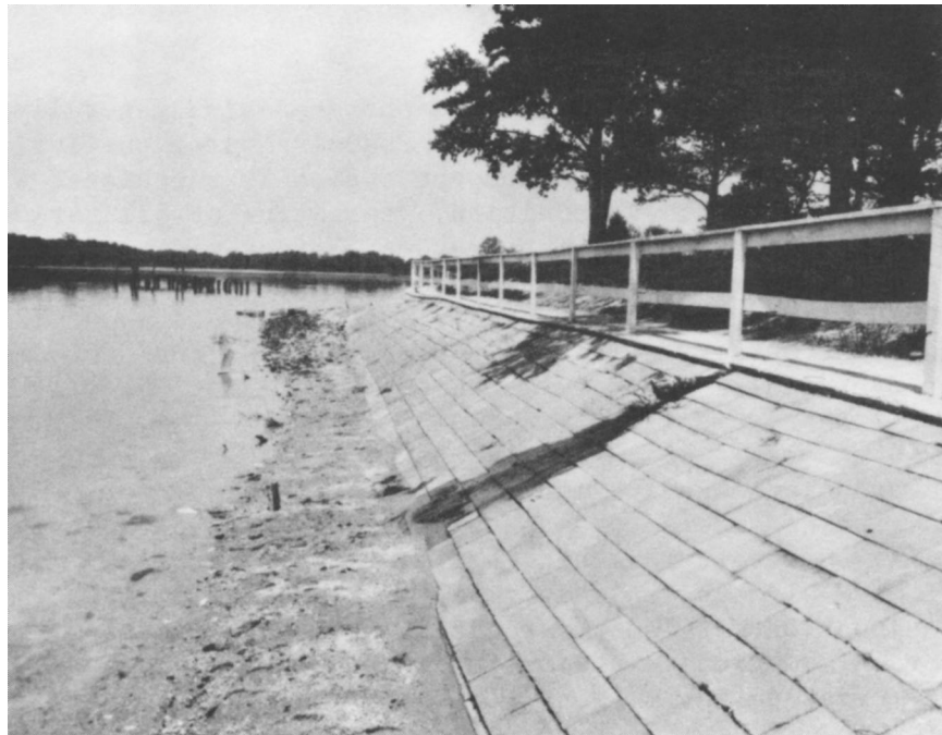
b. Erosion control structure (Maryland)
