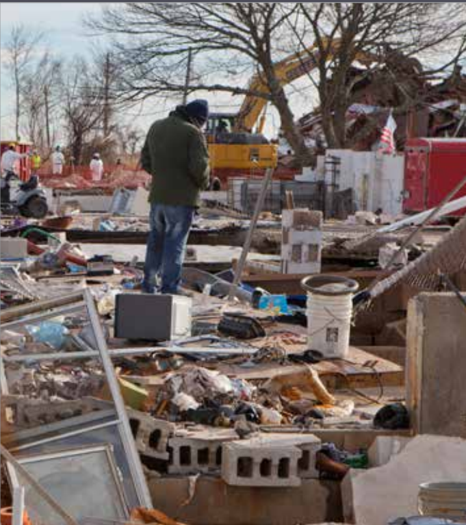
Residents of a Staten Island neighborhood look at properties destroyed by Hurricane Sandy. Homes will be removed because they are blocking street access. (Andrea Booher/FEMA)
