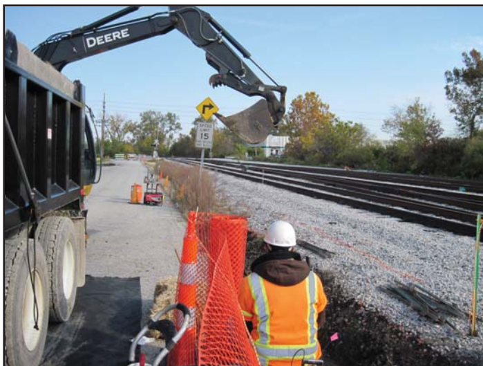
St. Louis North Country Vicinity Property 16 and Eva Load Out Area-3
