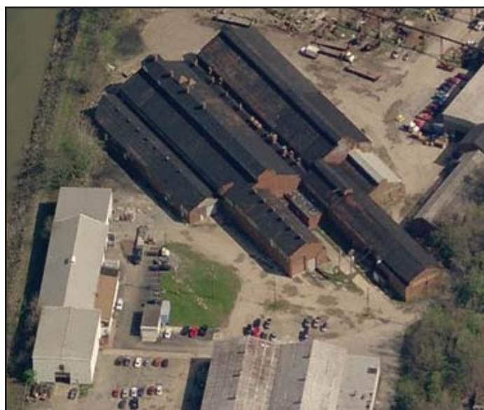
Superior Steel Site
