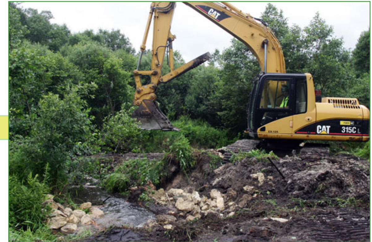
An excavator operator from a Wisconsin Department of Natural Resources crew reworks an embankment at Stillwell Creek on Fort McCoy's South Post. Stream biological monitoring, otherwise known as biomonitoring, was used to help determine where work needs to be done. (Photo by Scott T. Sturkol)
