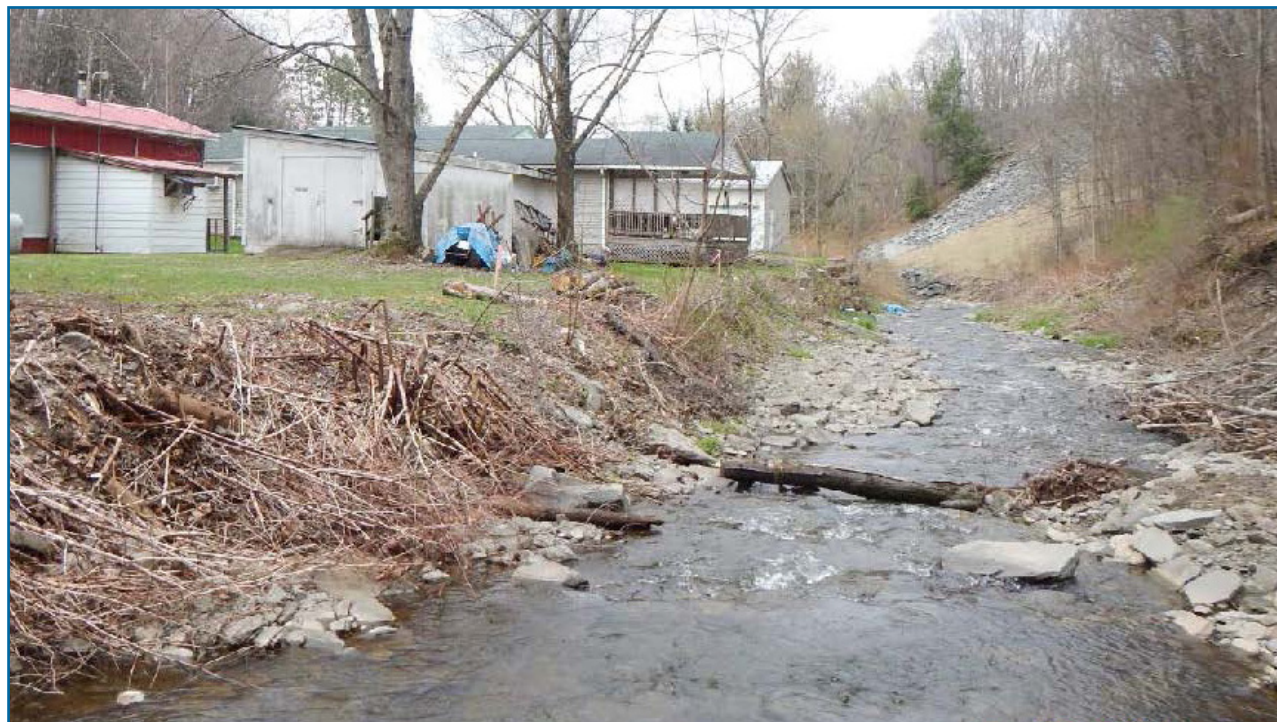
Third Brook today is now stabilized with large rock at the toe of the banks and native plant vegetation. (Photo by JoAnne Castagna) LEFT: Third Brook in May 2014 highly susceptible to failure after a major flood. (Photo courtesy Delaware County Soil and Water Conservation District)
