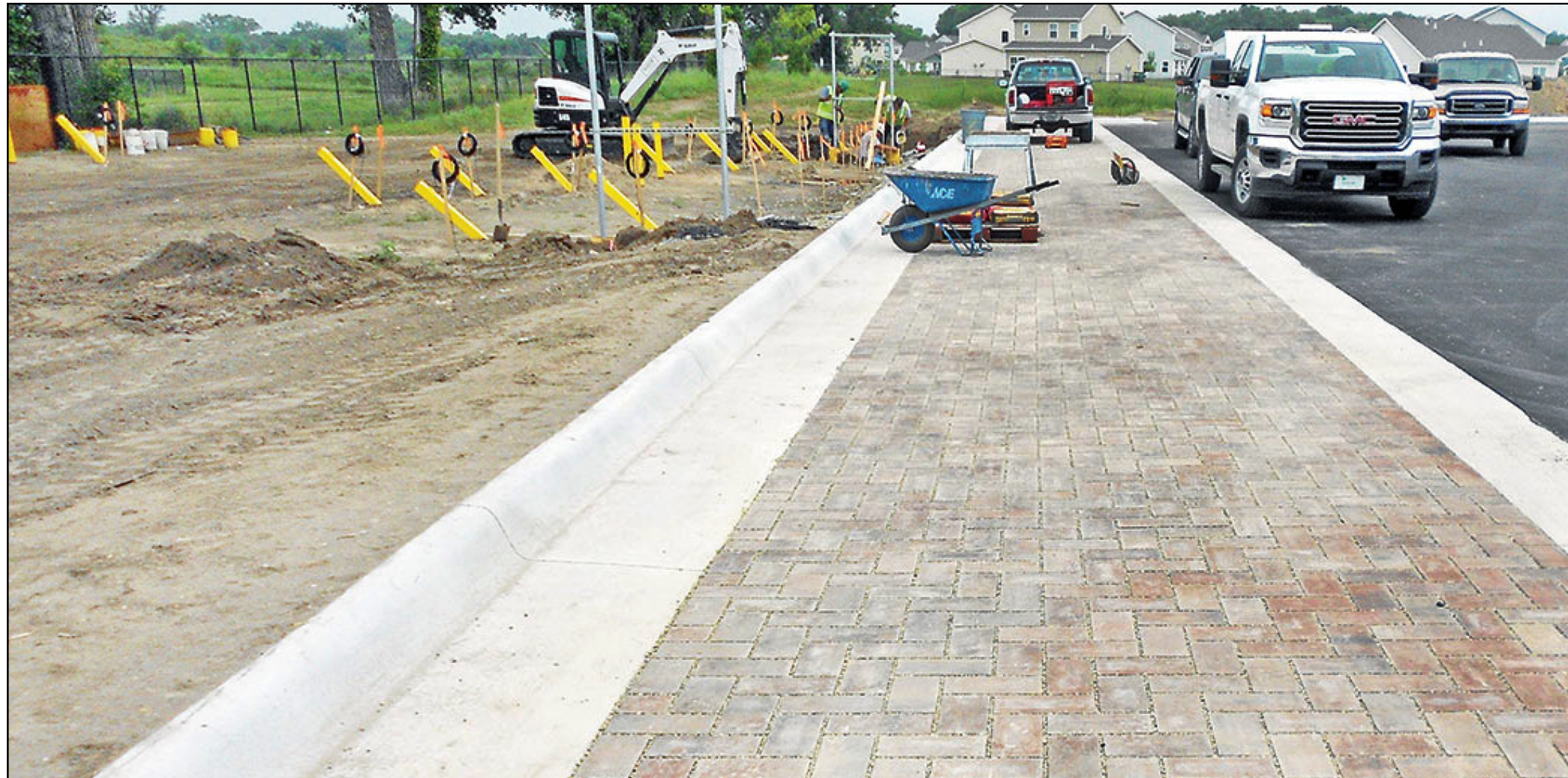
ABOVE: Shown under construction at Seitz Elementary School is the trench in which containers and sensors will sit. The containers will receive excess water from the parking lot. LEFT: Rain water will drain into this section of the parking lot, which features interlocking concrete pavement resembling bricks. (Courtesy photos)
