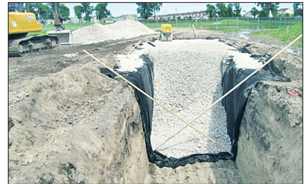
ABOVE: Shown under construction at Seitz Elementary School is the trench in which containers and sensors will sit. The containers will receive excess water from the parking lot. LEFT: Rain water will drain into this section of the parking lot, which features interlocking concrete pavement resembling bricks. (Courtesy photos)
