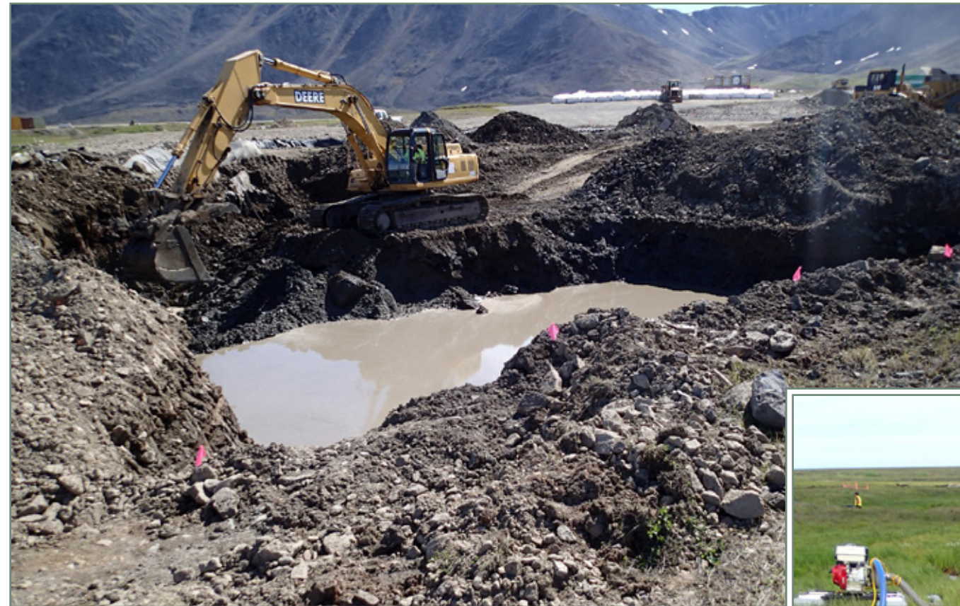
LEFT: Groundwater accumulated during soil excavation activities at the main operations complex for the Northeast Cape FUDS site in Alaska. In the background of the photo is Kangukhsam Mountain. BELOW: Bristol employees Johnny Willis and Albert Kulowiya operate the sediment suction dredge (top left) to remove loose sediment from the wetland. Sediment/water slurry was pumped upslope, flocculant added, transferred to geotextile tubes for dewatering, and excess water treated with GAC units before discharge to ground surface. (Photos by J. Craner)
