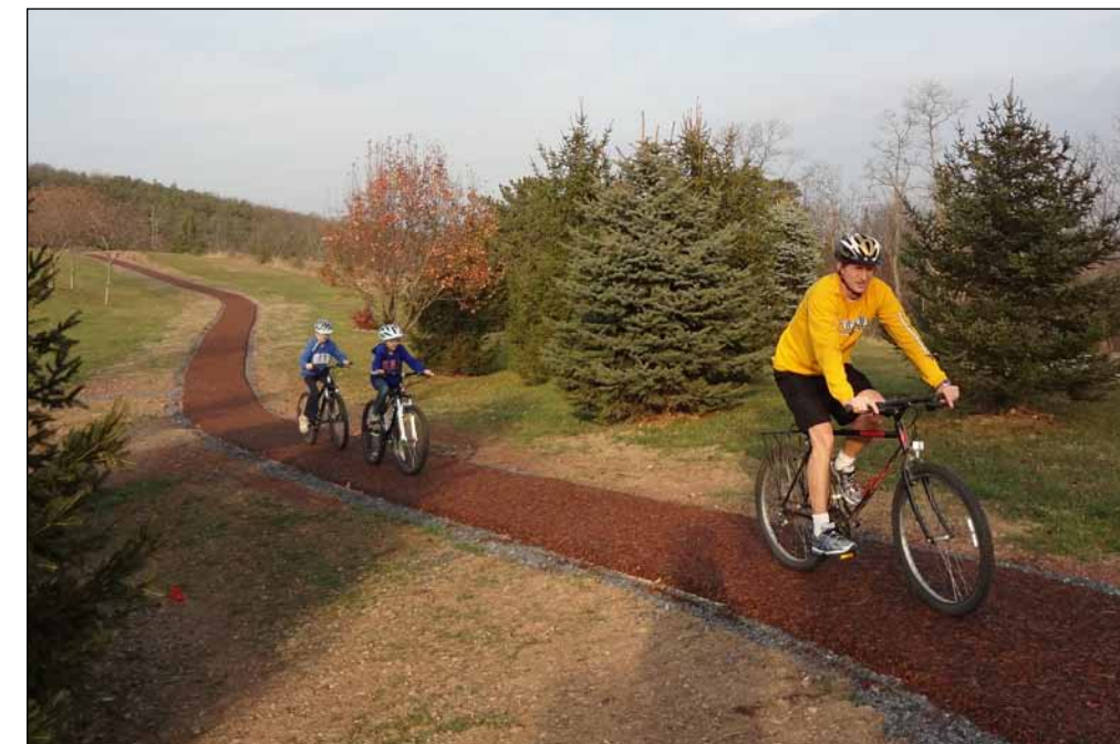
A family takes a ride on Raystown Lake's 2.3-mile Greenside Pathway around the Seven Points Recreation Area. The pathway, made entirely of recycled materials, reduces traffic congestion, increases pedestrian safety and provides a healthy alternative to driving.
