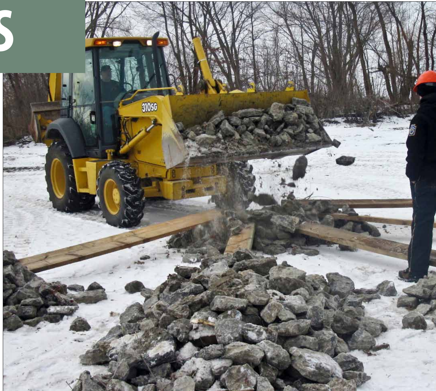
Shenango River Lake Maintenance Mechanic Ed Durch builds the middle rubble hump on a rock star to hold the boards in place. The staff at the U.S. Army Corps of Engineers Pittsburgh District lake and two employees from the Pennsylvania Fish and Boat Commission's Division of Habitat Management completed a two-day fish habitat improvement project in February. The cost-sharing program enabled both agencies to supply materials, manpower and expertise. The project focused on building rock stars and rock rubble humps in the small cove just east of the marina, and the southern and eastern shorelines of the old Mercer Recreation Area. Rubble humps on a point adjacent to the cove where the rock stars were constructed will act as a deep water staging area for fish in the spring before they spawn in the shallows. Since rubble humps are traditionally placed on flats or shoals in reservoirs, the best placement occurs during winter drawdown with heavy machinery. Both types of structures will improve fishing for bank and boat anglers. The structures provide forage type habitats for invertebrates, crustaceans and baitfish, and attract walleye, black bass and panfish. (Photo by Kyle Kraynak, Shenango Lake park ranger) See more photos at www.flickr.com/photos/pittsburghcorps/ .
