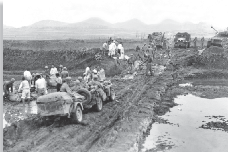
A jeep and trailer move across a temporary earthen bridge that is being reinforced with sandbags Engineer School, 83-56-2
