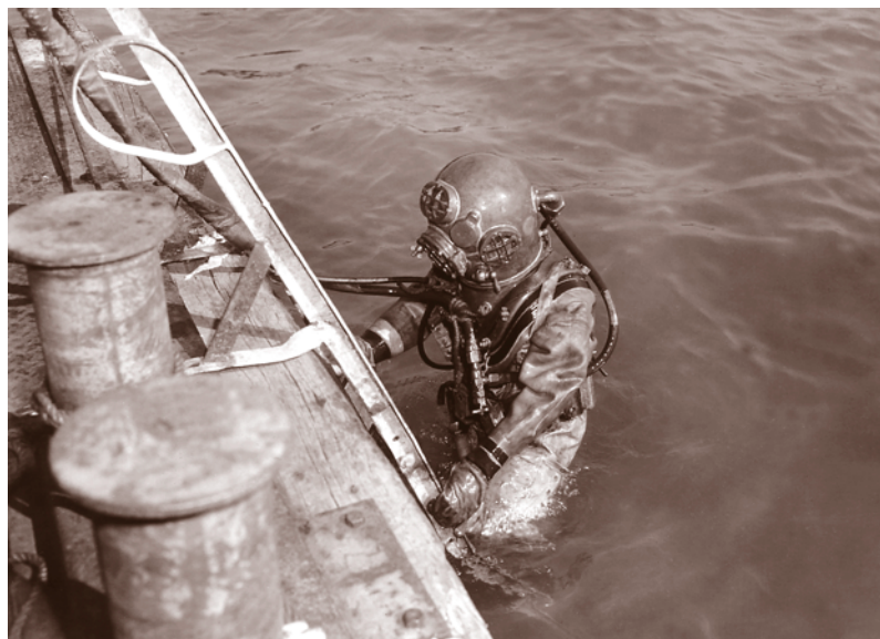
MSgt. Melvin Alderman of the 50th Engineer Port Construction Company slowly climbs aboard the support barge after a dive RG 111, SC-451590
