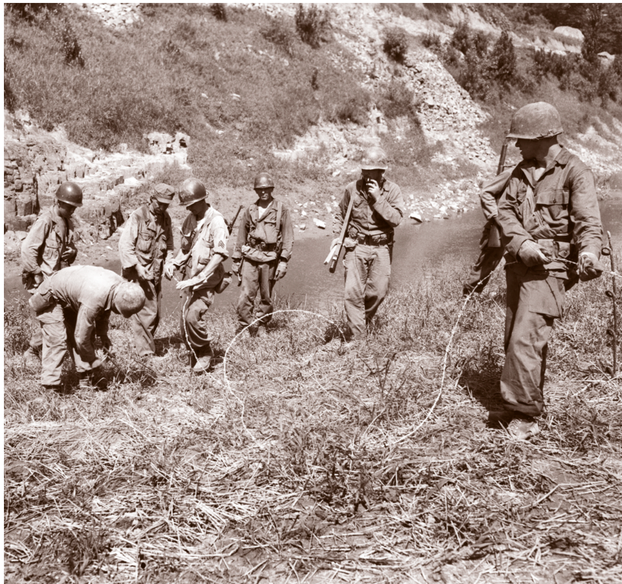
Soldiers of the 14th Engineer Battalion place a barbed wire entanglement on the banks of the Naktong River, 10 August 1950 Engineer School, Korea 011
