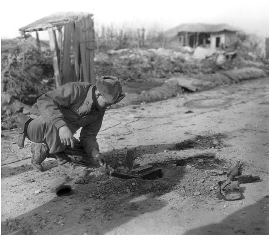
Second Lt. John Kane, 65th Engineer Battalion, removes a Chinese box mine RG 111, SC-357543
