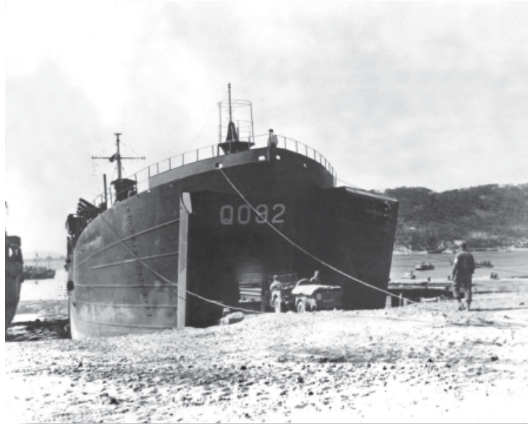
A jeep and trailer are loaded into an LST Engineer School, 30-10-20
