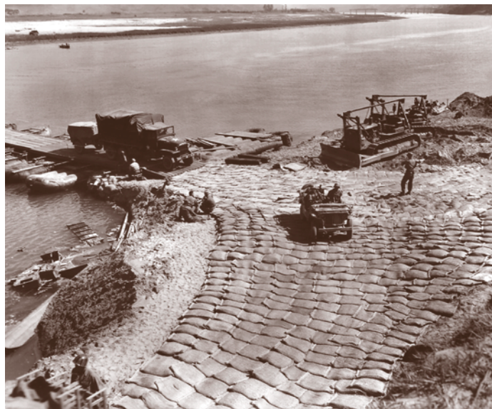
Engineers use rice bags to stabilize the roadbed near a ponton bridge RG 111, SC-349361
