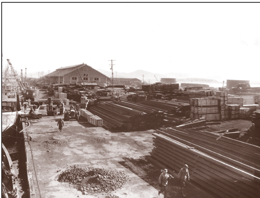
Engineer supplies stored on the pier at Inch'on RG 111, SC-354721
