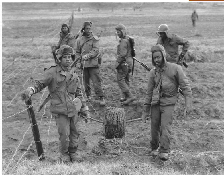
Engineers of the 77th Combat Engineer Battalion lay a single-apron barbed wire fence RG 111, SC-359427
