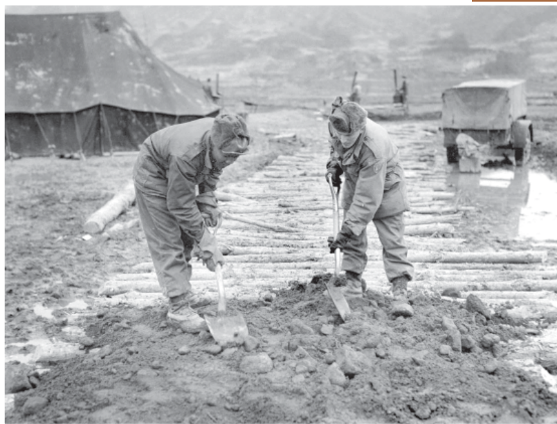
In the midst of the spring thaw, engineers lay dirt and rocks over a corduroy road to enable supplies to reach the mess hall Engineer School, 13-14-1
