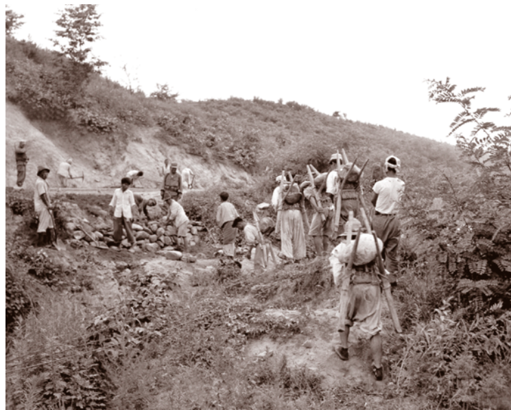
Korean laborers use A-frame packs to carry stone for the construction of a revetment near Yonchon, July 1951 Engineer School, 93-66-6
