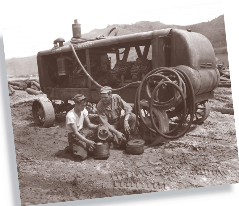
Members of the 84th Engineer Construction Battalion change the oil and clean the filters on an air compressor RG 111, SC-379254
