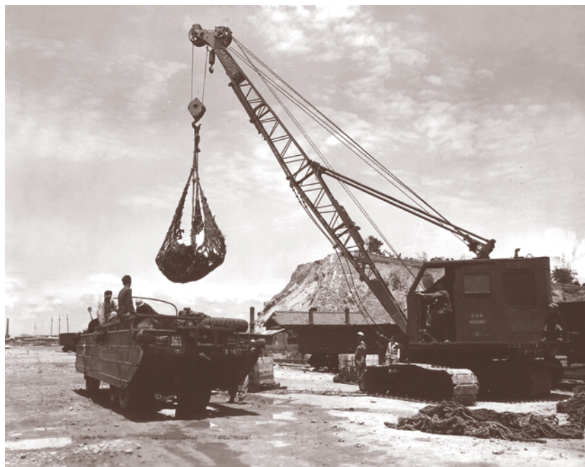
Engineers of the 532d EB & SR transfer 155 mm artillery shells from a DUKW to a waiting railroad car RG 111, SC-370368
