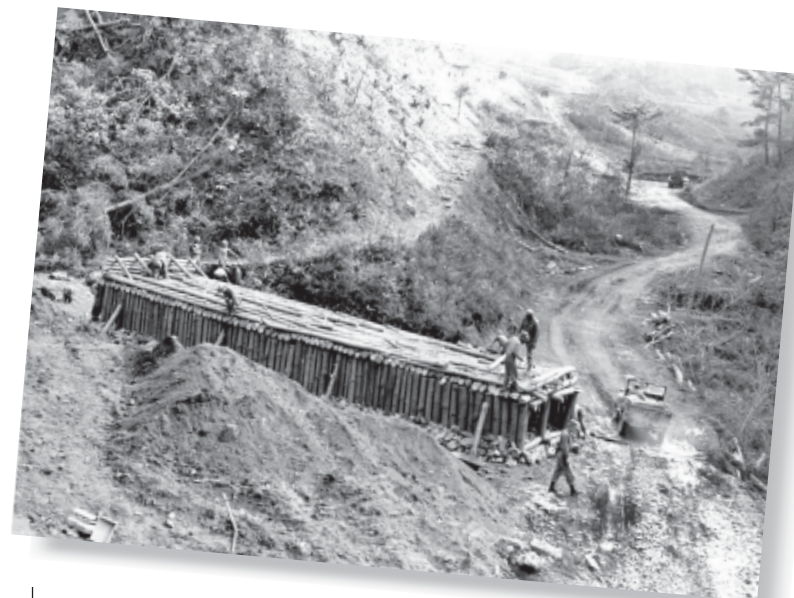
U.S. and Korean engineers construct a timber culvert during the construction of a new road, October 1951 Engineer School, Korea-081
