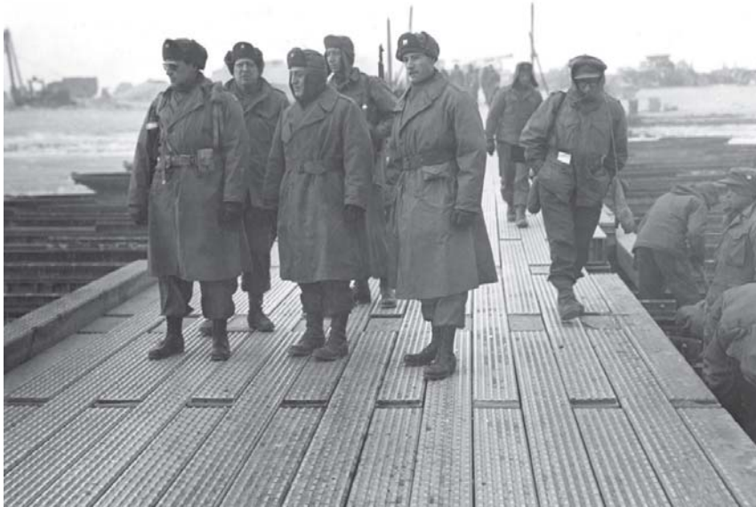
After the last UN forces withdrew from Seoul, Lt. Gen Matthew Ridgway (front row, left) and Col. Emerson Itschner (front row, center) gave the order to dismantle the bridge and destroy those sections that could not be quickly removed, 4 January 1951 Engineer School, 42-6-56
