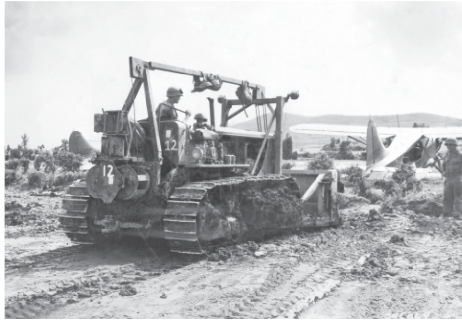
A bulldozer strips and does rough grading on a forward airstrip designed to accommodate reconnaissance, supply, and evacuation aircraft Engineer School, 11-13-5
