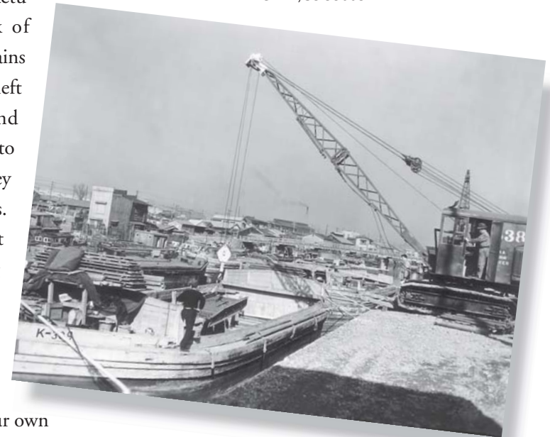
Treads for a Bailey bridge are loaded on a barge at the Yokohama Engineer Depot, 28 January 1951 RG 111, SC-356681
