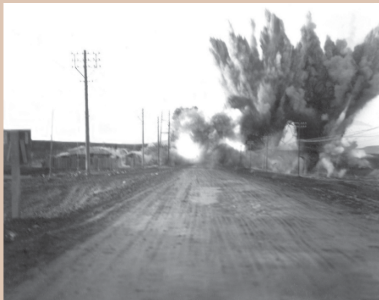
Engineers destroy a railroad bridge near Hamhung to slow the enemy advance Engineer School, 71-19-8
