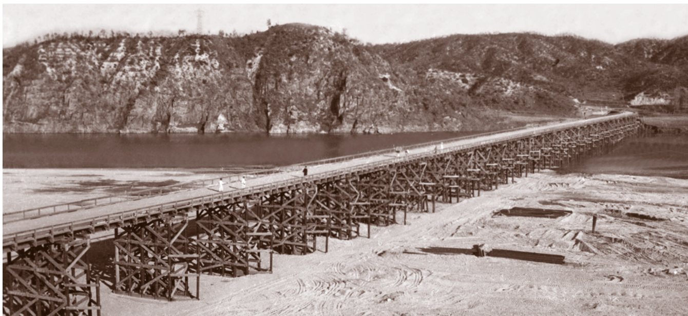
Yoju Bridge, August 1951 Engineer School, 41-1-129
