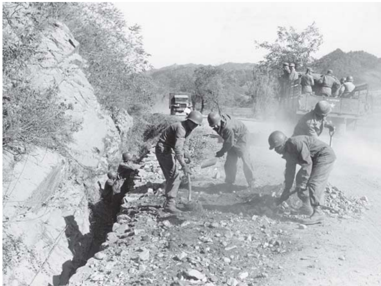
Using hand tools, soldiers of the 65th Engineer Battalion work to fill holes in the road near Hagammyond, Korea Engineer School, Korea 86
