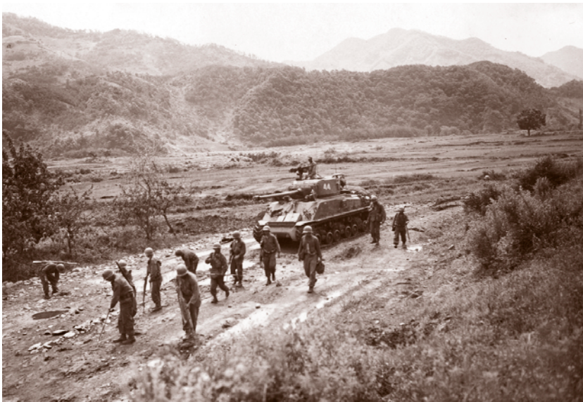
Soldiers sweeping the road for mines before an advancing M-4 tank Engineer School, 119-13-1
