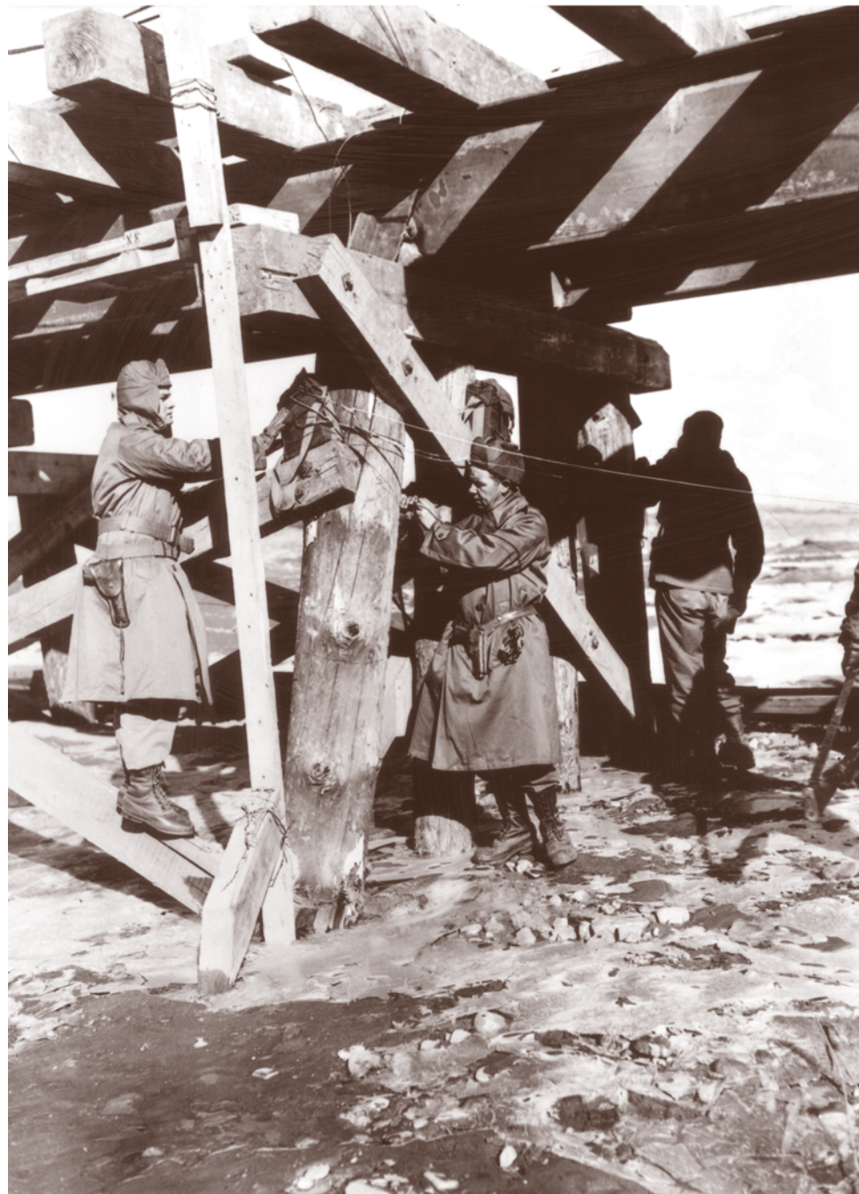
Engineers place satchel charges on a railroad bridge near Pyongyang prior to demolishing it RG 111, SC-355302
