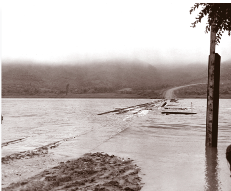
A section of the Spoonbill Bridge is covered by flood waters of the Imjin River, July 1953 Engineer School, 43-6-5
