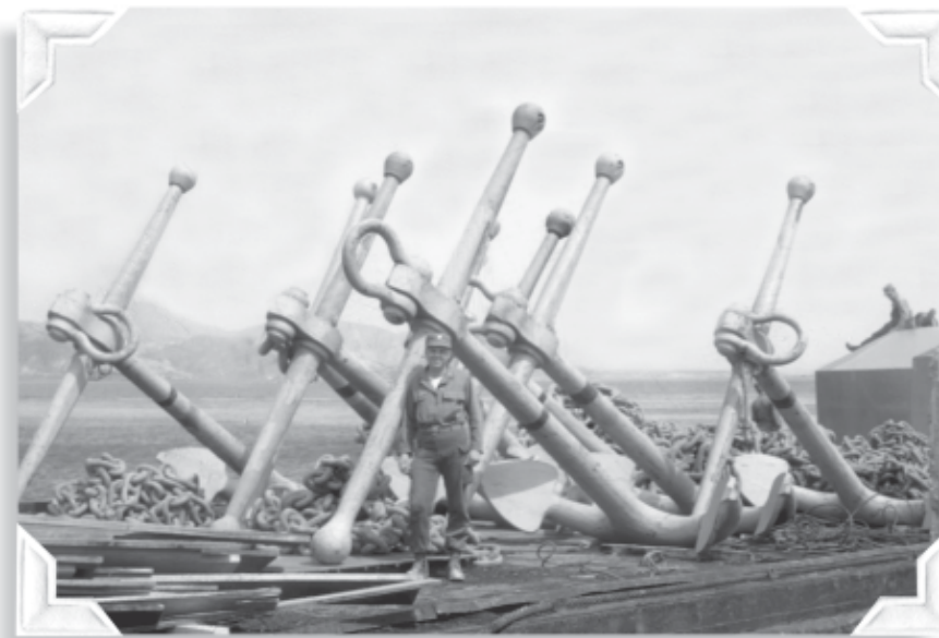
Mooring anchors waiting to be placed at the offshore fuel terminals Gray Collection
