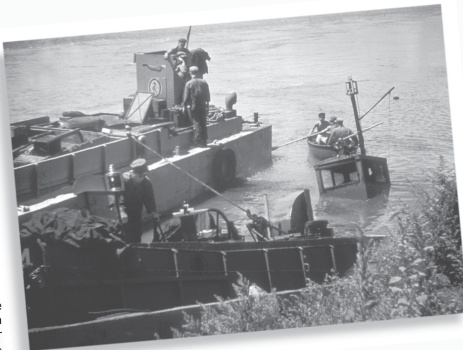
Engineers raise an LCM sunken in the Han River Roberts Collection
