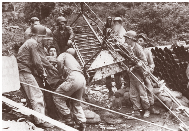
Men of the 31st Infantry Regiment and 13th Engineer Battalion evacuate a wounded soldier using an aerial tramway Engineer School, 148-16-164
