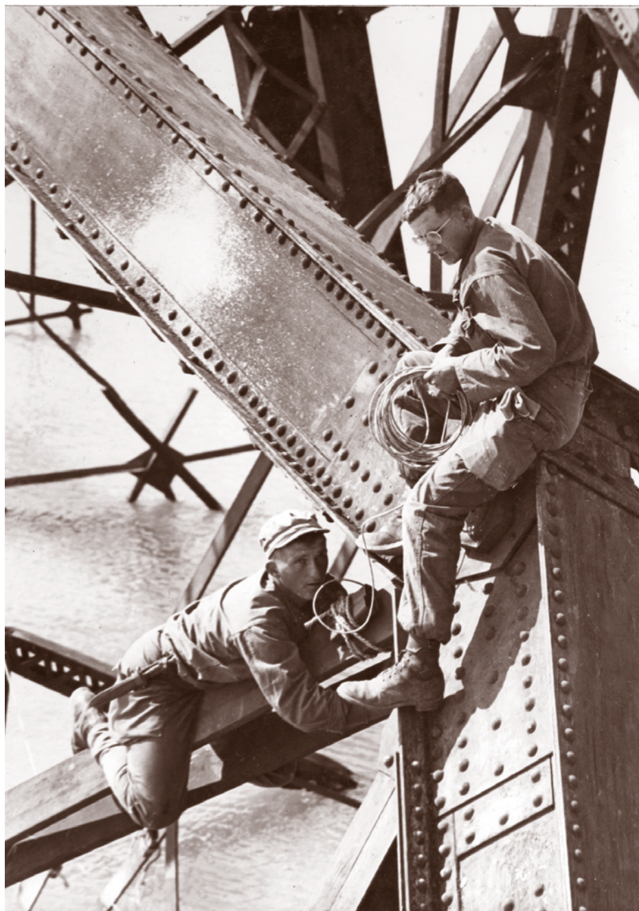
Engineers place explosive charges to demolish a damaged bridge on the Naktong River Engineer School, 71-19-37
