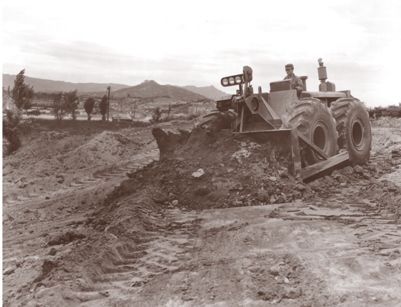
Engineers experiment with a newly received Tournadozer at a facility near Seoul RG 111, SC-378098
