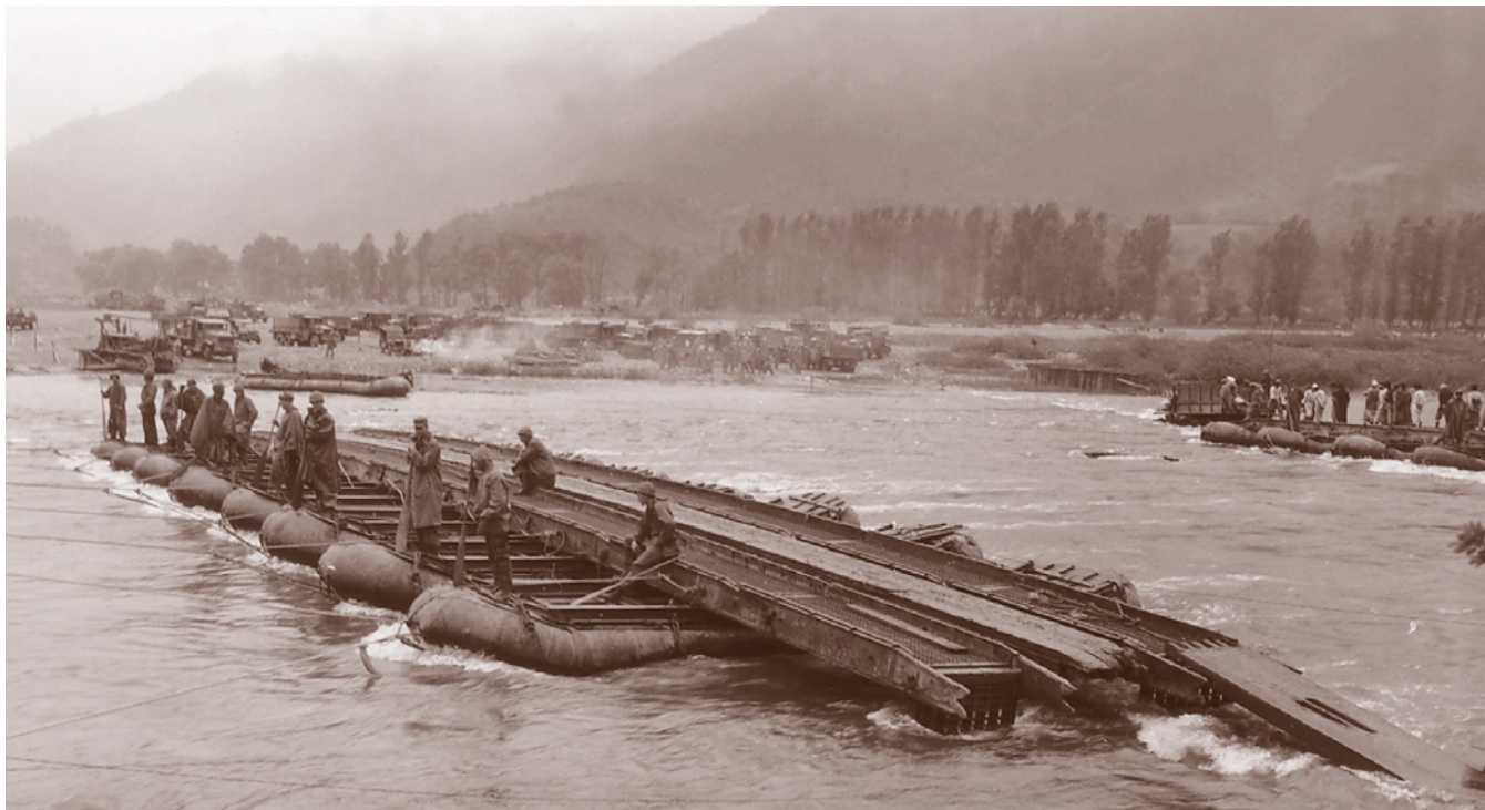
Men of the 185th Combat Battalion stand watch over a bridge damaged by floodwaters on the Soyang River, May 1951 RG 111, SC-369385
