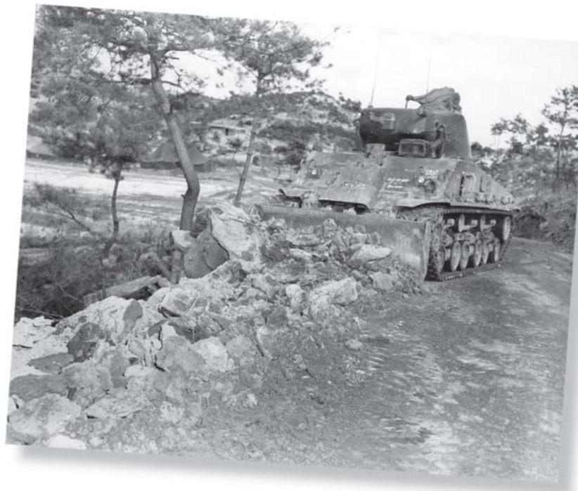
A tank dozer clears a road in western Korea Engineer School, 92-62-6
