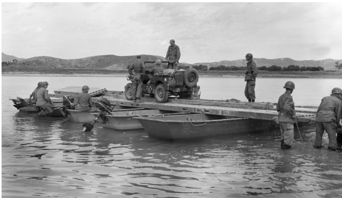
Members of the 3d Engineer Battalion ferrying a jeep across the Naktong River Engineer School, 30-25-100
