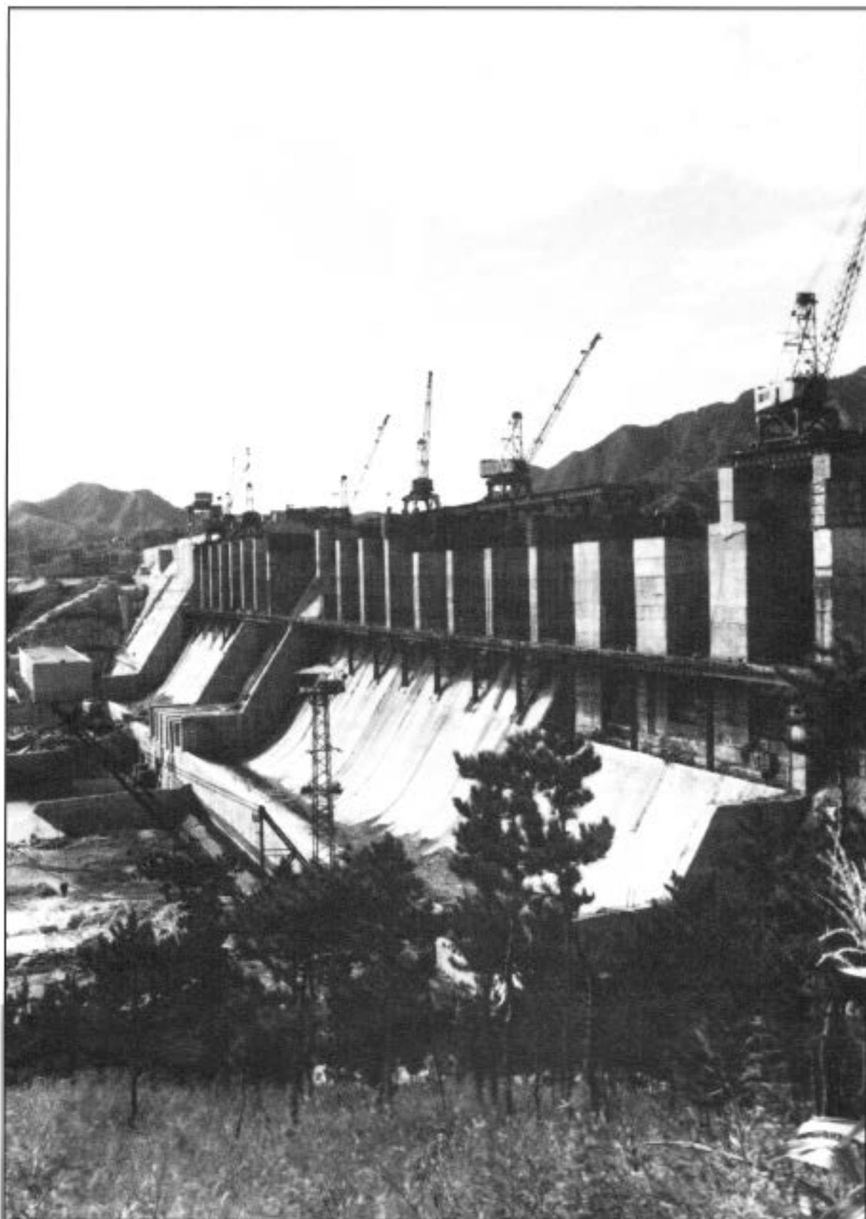
The dam at the Panjiakou Power Station during General Morris' trip to China in early 1980.
