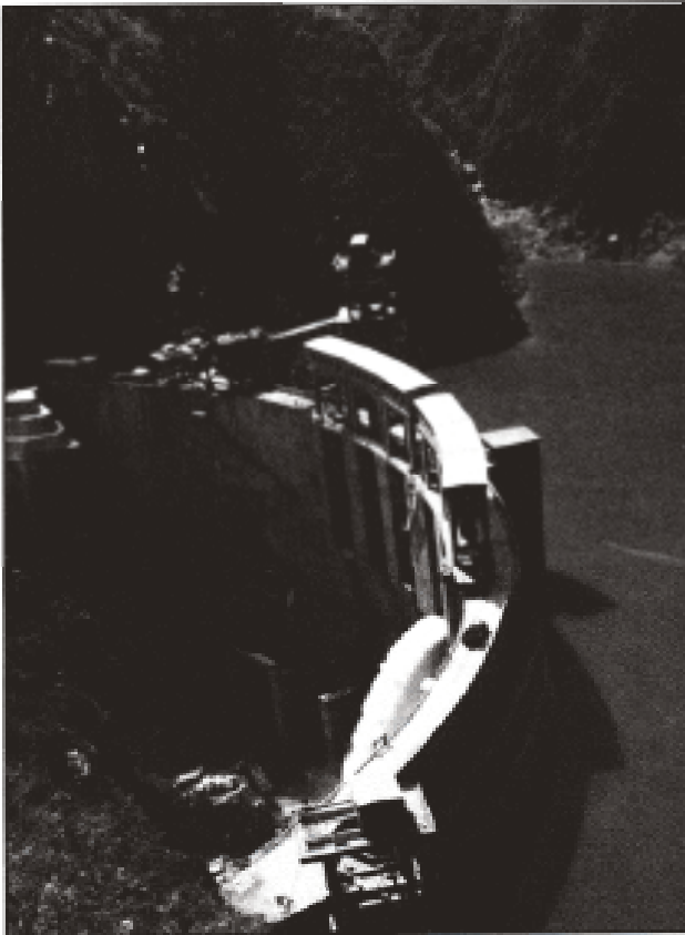
The dam at the Shimen Power Station during General Morris' trip to China in 1980.
