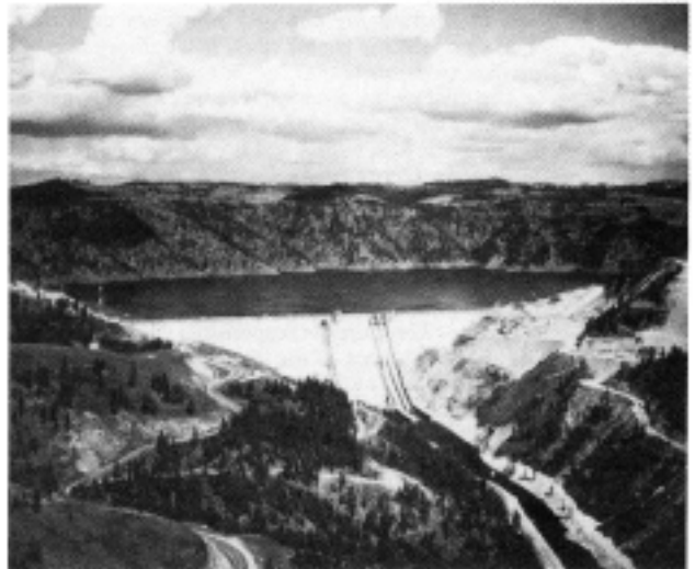
The power-generating capacity of the multipurpose Dworshak Dam in Idaho is currently being expanded
