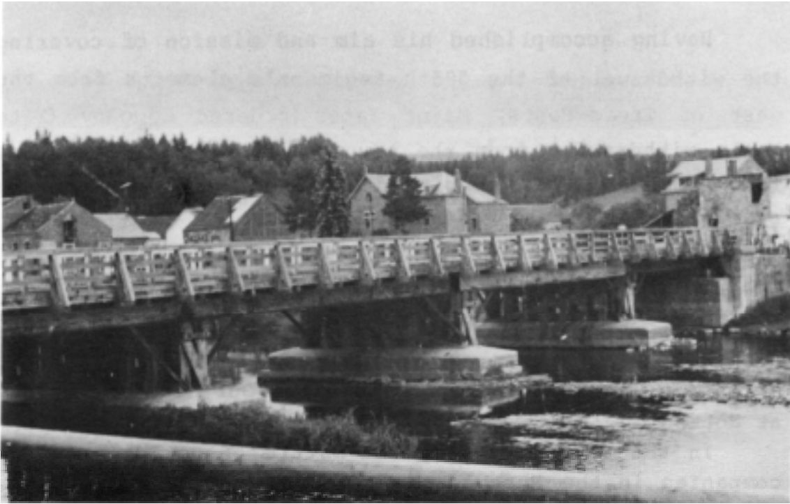
The vital Ourthe River bridge at Hotton
