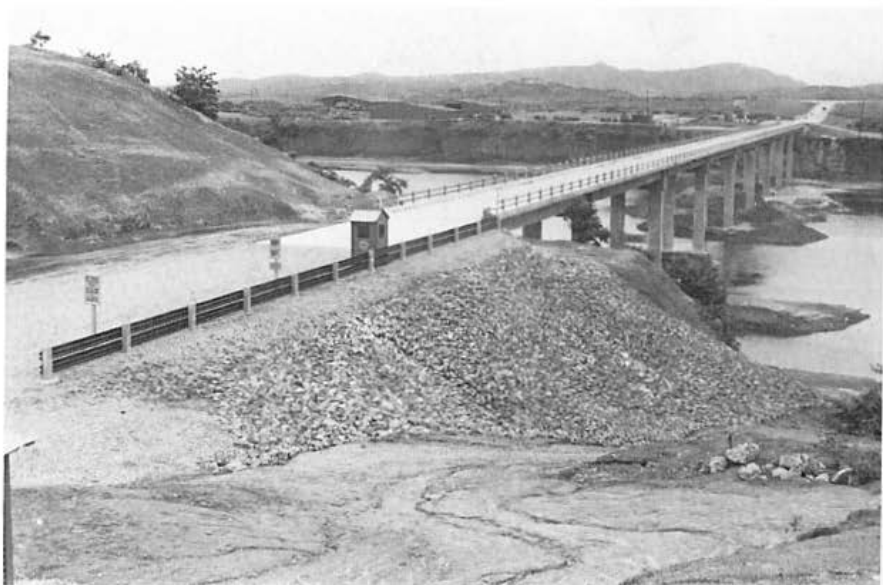
Figure 60. Completed Libby bridge from the west bank on 4 July 1953.
