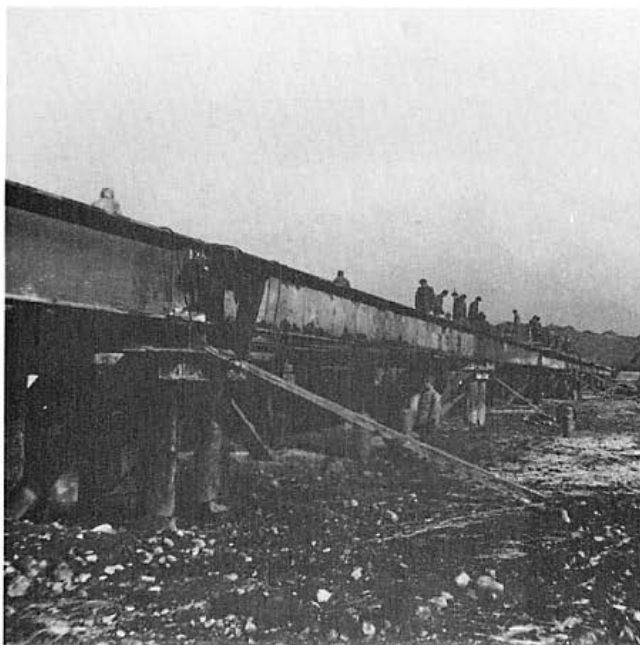
Figure 29. Troops placing decking from pier 16 to the north abutment. This was the only span which used six 24-inch girders. Note angle-iron diaphragming between girders. Visible at center is two-inch by six-inch laminated sub-decking and beyond that is three-inch by twelve-inch diagonal decking.
