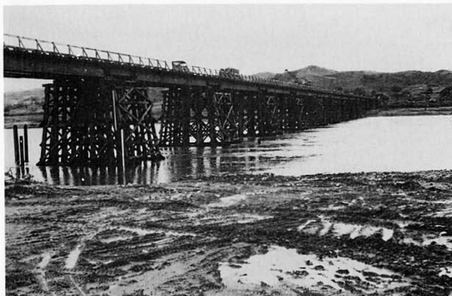
Figure 9. The high-level Pintail bridge on 27 July 1952, just three days after the 62d Engineer Construction Battalion had opened it.
