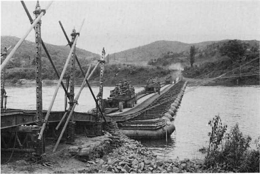
Figure 3. Artillerymen of the 1st Cavalry Division crossing the floating treadway bridge at the Whistler site in early August 1951.
