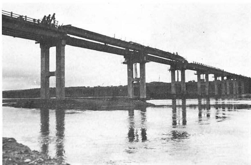
Figure 55. Chain hoist lowering girder complete with sub-decking across piers 7, 6, and 5.
