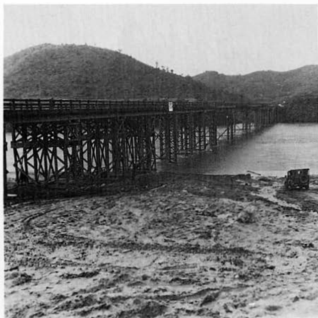
Figure 10. The high-level White-front bridge on 27 July 1952.
