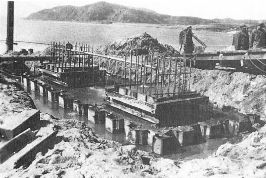
Figure 41. Cofferdam 3 filled with 240 cubic yards of concrete constituting the initial or A pour. Water is being used to cure the concrete, and the scaffold floor at right is ready to be set in place.
