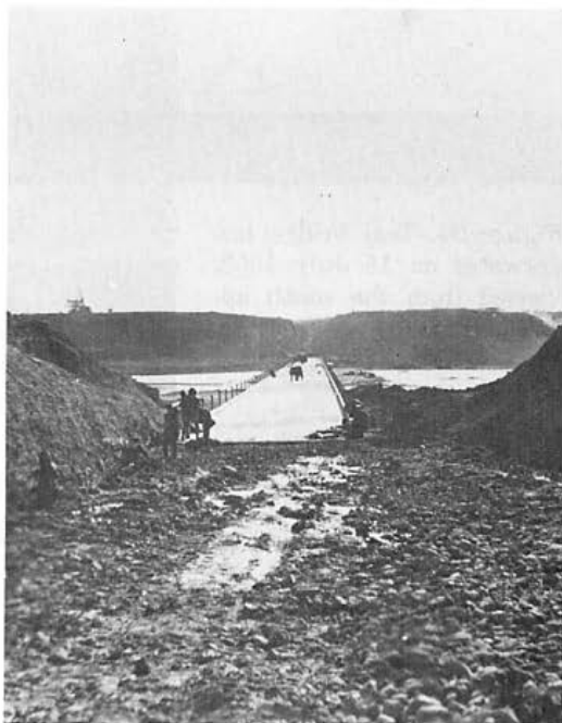
Figure 32. Teal bridge from the north shore on 16 January 1953 when almost completed. This view shows the removable guardrail.
