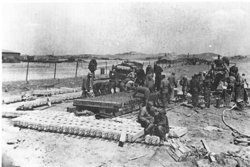
Figure 49. Soldiers casting guardrail posts. The reusable forms shown could cast batches of 66 posts at once.
