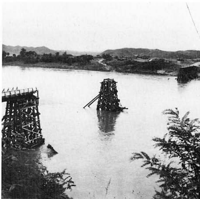
Figure 15. The high-level Teal bridge after the flood of 24-25 August 1952.
