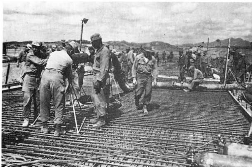
Figure 57. Troops setting up the pumpcrete pipe to pour concrete decking.
