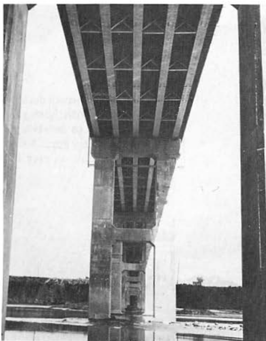
Figure 61. View looking east at the completed piers and superstructure of Libby bridge.
