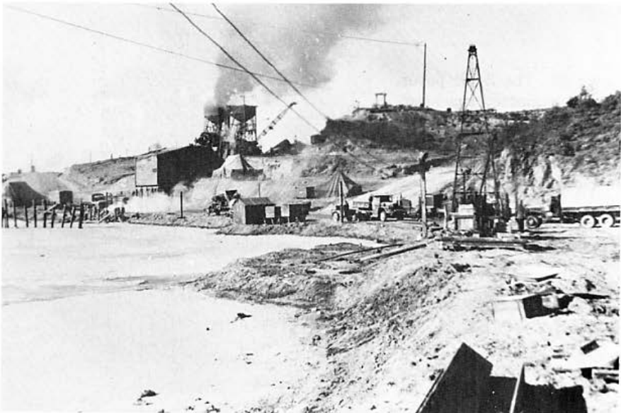
Figure 43. The central concrete batch plant, which furnished hot aggregates or warm concrete from its location on the Imjin's west bank. The plant's two 60-ton bins fed coarse and fine aggregate to the 80- to 150-ton-per-hour dryer that discharged into bins inside the plant.
