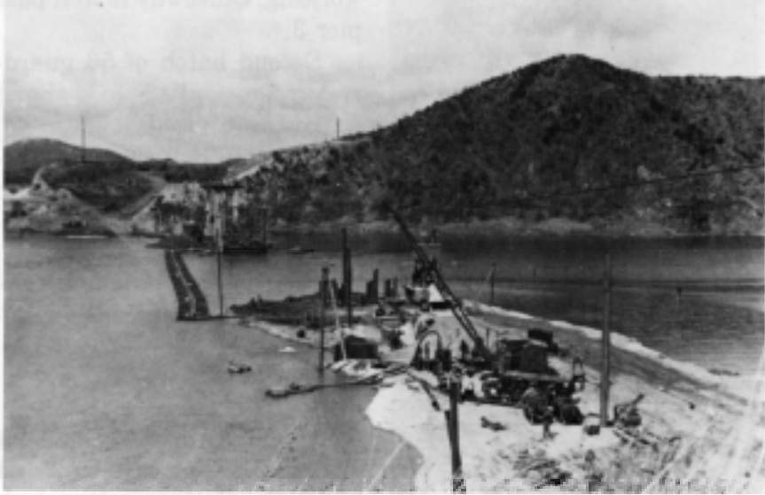
Figure 70. View of the footbridge that enabled the pumpcrete machine to pump concrete from its location near pier 3, at center, to pier 6 across the river channel.
