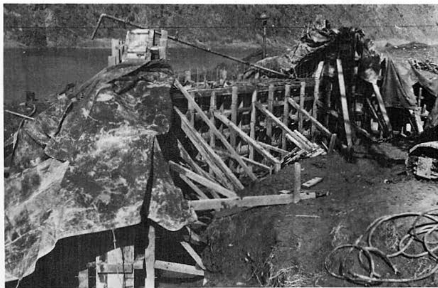
Figure 68. East abutment, completed on 25 March 1953, prior to stripping of forms.
