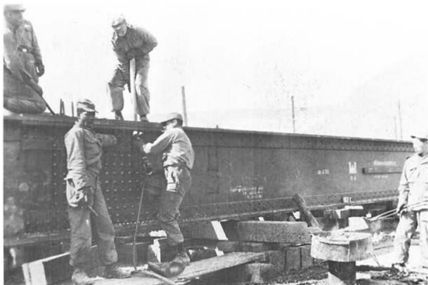
Figure 51. Riveters at work on steel beams. Newly trained American and Korean riveters developed their skills so quickly that a 121-foot span was launched with a deflection of only 17 inches.
