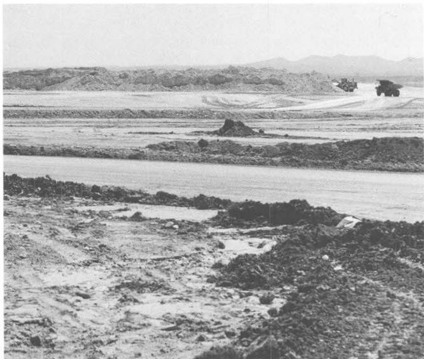
Excavation of Glide Path Hill at Ramon
