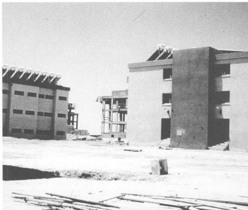
Airmen's dormitories, with solar panels on rooftops, at Ovda.
