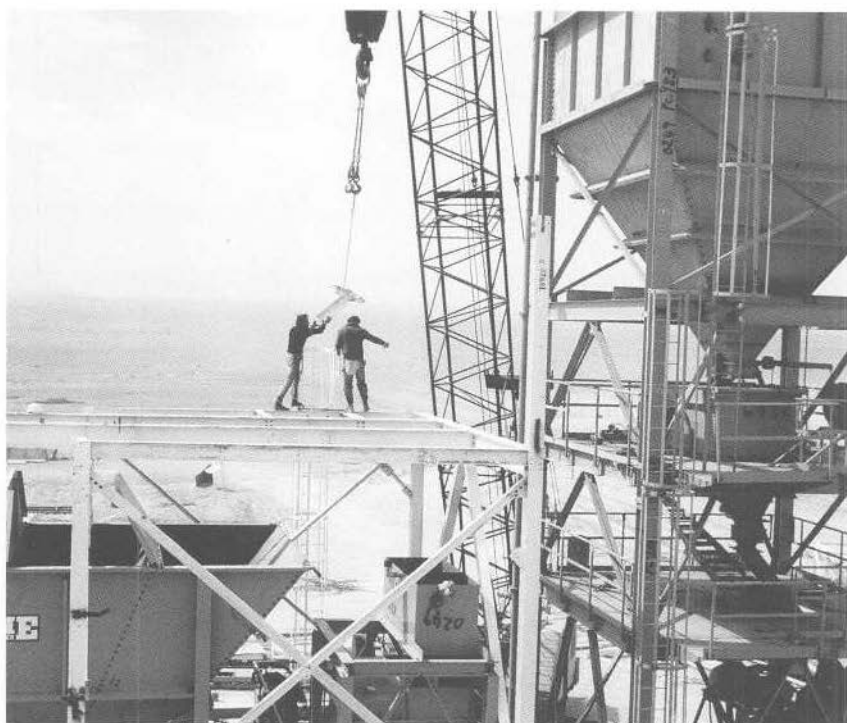
Bulk cement storage facility under construction at Ovda in the spring of 1980.
