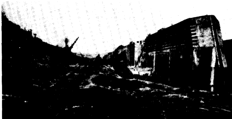
The Large Lock under Construction
