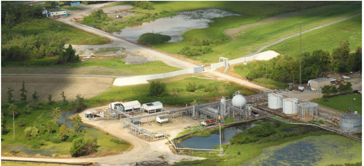
Above: Aerial image of Goodhope Floodwall. Image taken July 2012.
