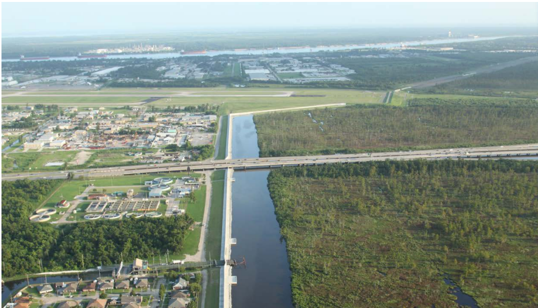
Aerial image taken in July 2012 of the completed West Return Floodwall.
