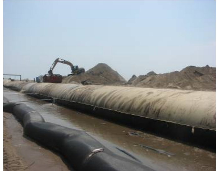
Geotextile Center Tube (white tube) and Anchor Tube (black tube)
