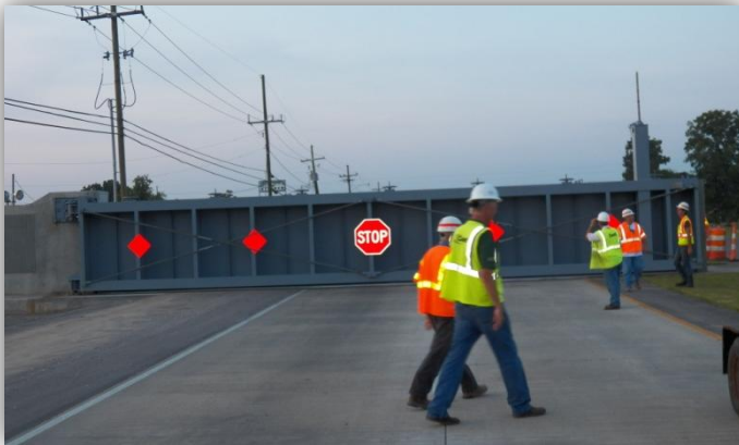
WBV-09c Closed Highway Swing Gate
