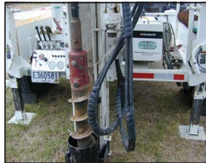
Installation of temporary monitoring wells at Dixon Tomato site
