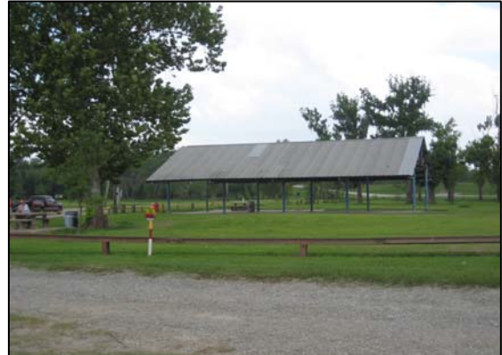
31 Photograph 2-5. U.S. 61 Recreation Area
