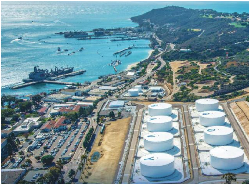
NAVSUP Fleet Logistics Center San Diego's Defense Fuel Support Point facility located on Naval Base Point Loma.
