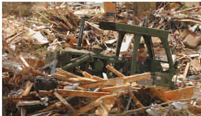
U.S. Army Guardsman Spc. James Meidl, heavy equipment operator, from the 890th Engineer Battalion, Columbia, Mississippi, operates a D-7 Dozer to help clear the roads while in Pass Christian, Mississippi, during humanitarian relief efforts in support of Joint Task Force Katrina, 4 September 2005. U.S. Air Force photo by Master Sgt. James M. Bowman.
