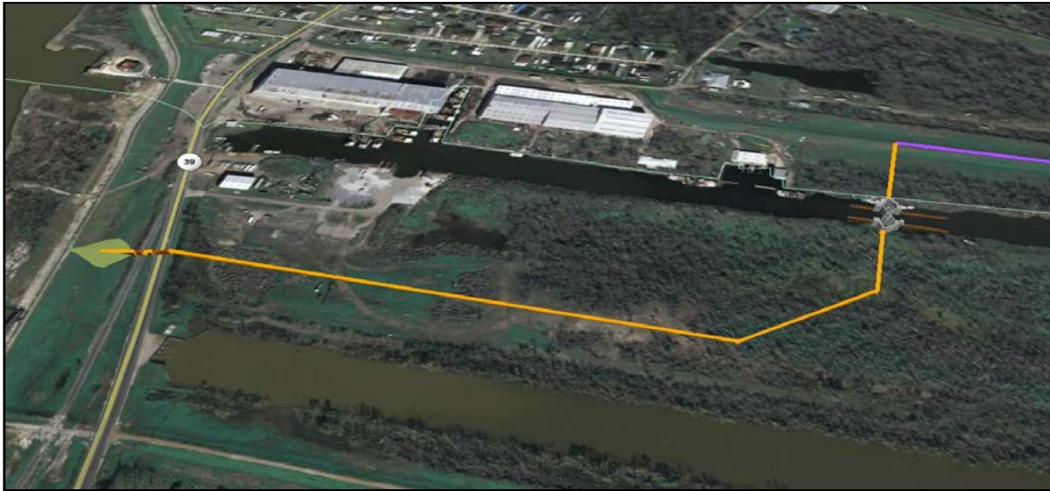
Figure 2.4. Aerial view of the Caernarvon Floodwall and Gate in St. Bernard and Plaquemines Parishes.
