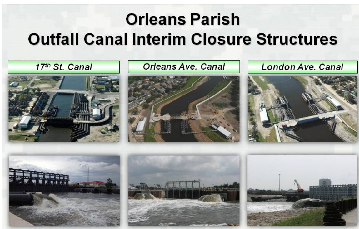
Figure 2.3. Interim Closure Structures. These temporary features provide the 100-year level of risk reduction at the mouths of the three outfall canals in Orleans Parish.
