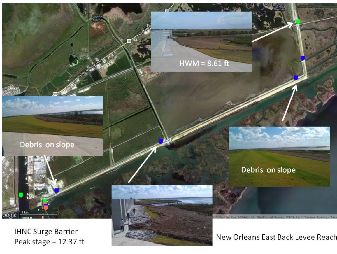
Figure 4.9 Damage assessment data from the New Orleans Back Levee Reach.
