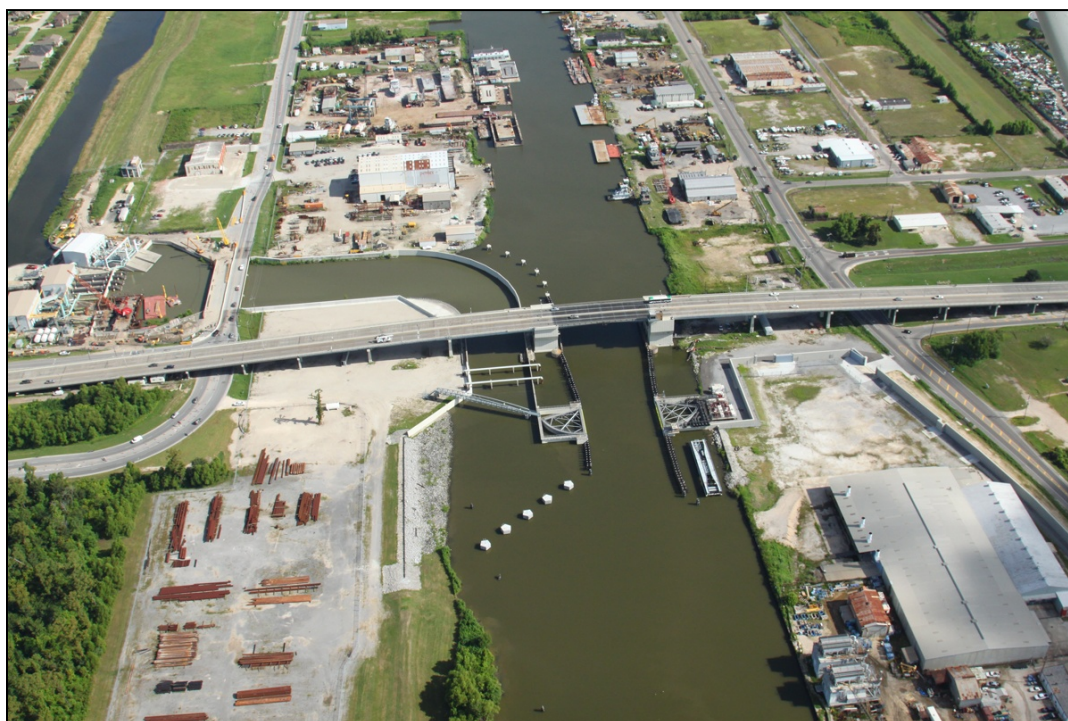
Figure 2.7 Aerial view of the Harvey Sector Gate on the Westbank in Jefferson Parish.
