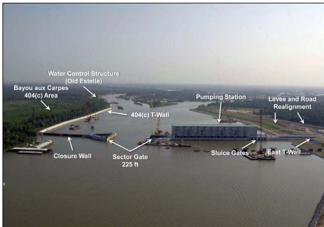
Figure 2.6. Aerial view of the West Closure Complex and Estelle Water Control Structure in Plaquemines and Jefferson Parishes.
