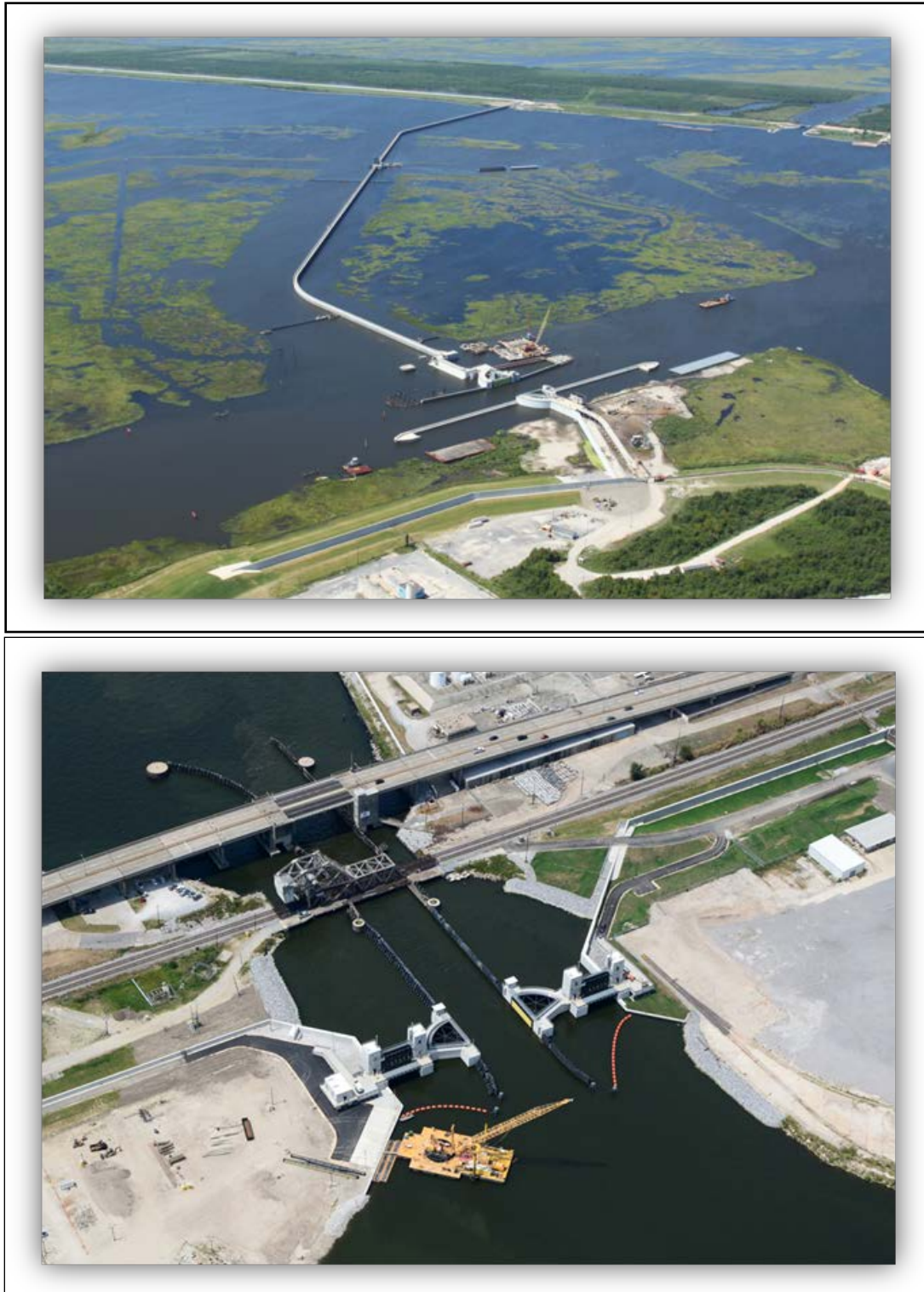
Figure 2.2. IHNC Surge Barrier (top) and Seabrook Complex (bottom) in Orleans and St. Bernard Parishes.
