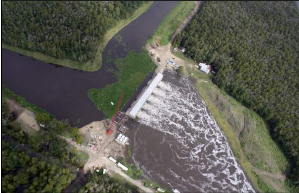
Figure 7.3.11 Aerial image of Marvin J. Braud Pump Station in Ascension Parish during normal operations.
