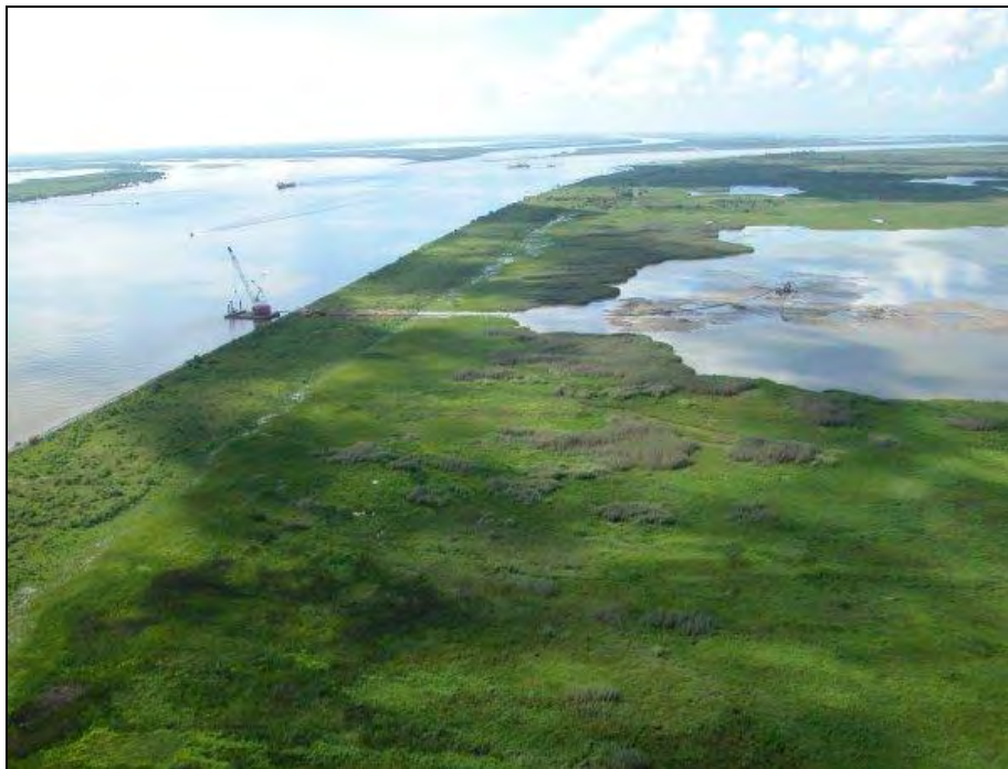
Figure 2-17. Dredge Piping Sediment from the Mississippi River to Restore Marsh
