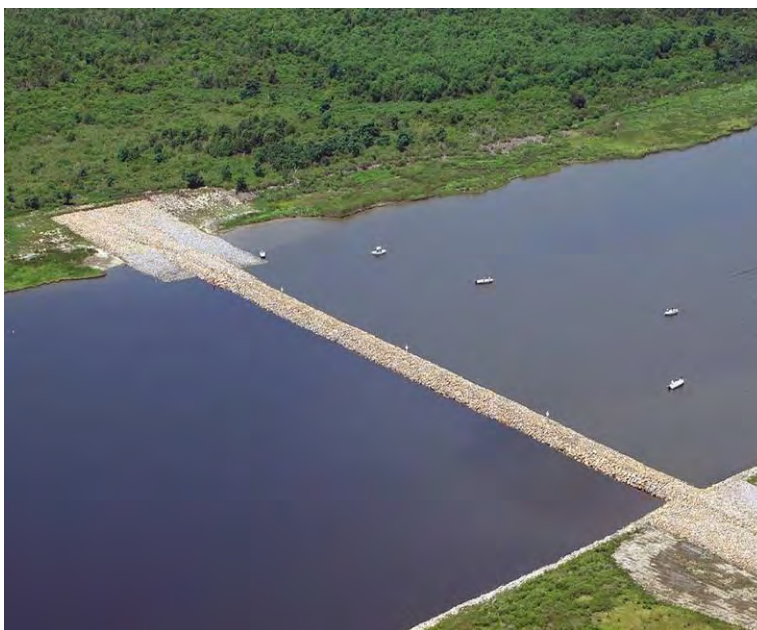
Figure 1-2. Completed MRGO Rock Closure Structure
