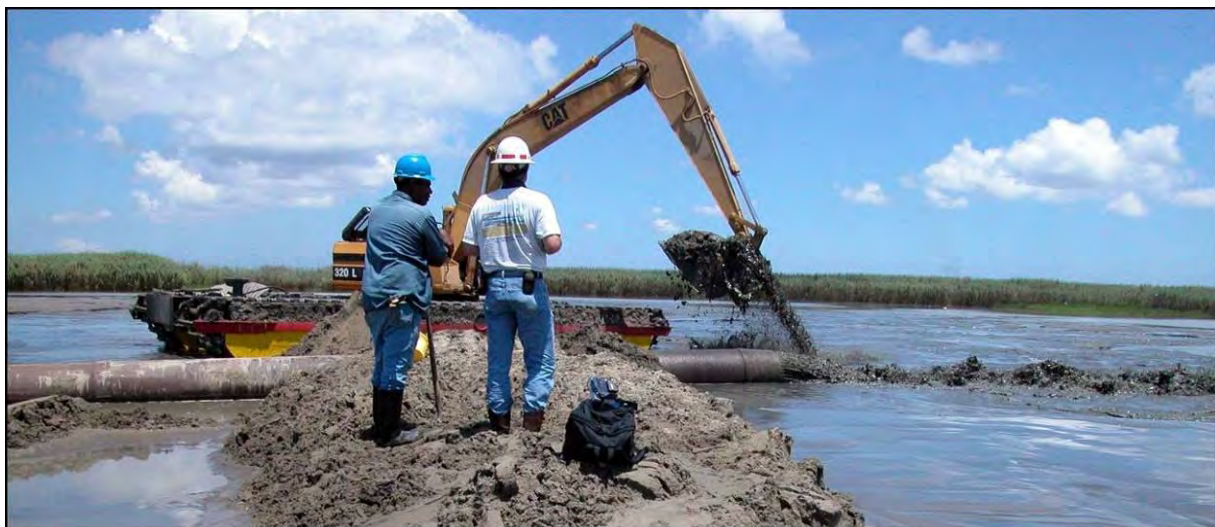
Figure 2-16. Dredge Material Placement for Marsh Restoration
