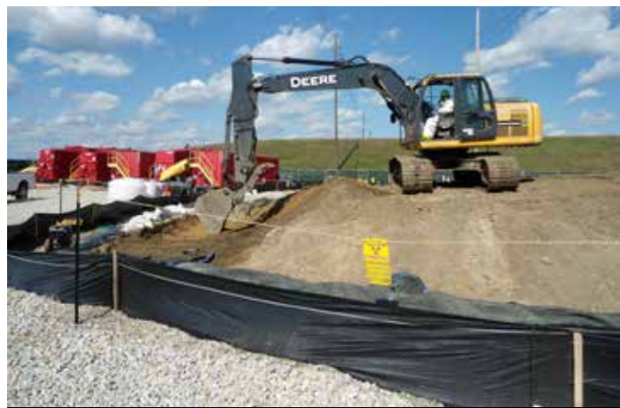
Excavation of AOC-6 at the DuPont Chambers Works
