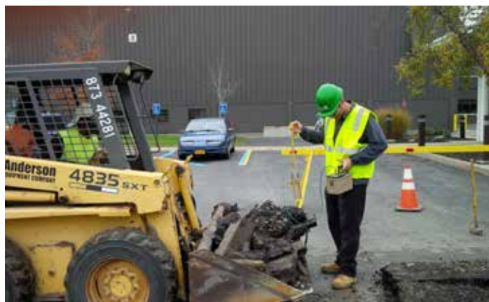
Linde Site monitoring well decommissioning during site restoration
