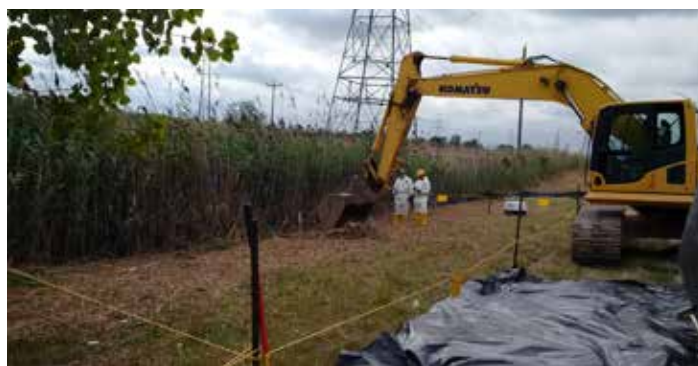
First scoop of soil removed during remediation of the Seaway Site Northside Area
