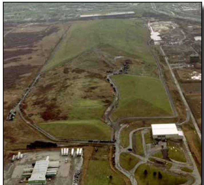
Seaway Site aerial photo, looking south
