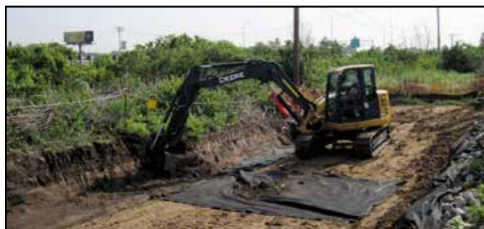
Loadout pad expansion at the St. Louis Airport Site
