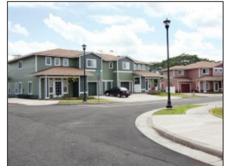
U.S. Army Garrison - Hawaii housing communities like Helemano Military Reservation, a housing area for Schofield Barracks, continue to expand the renewable energy program with the installation of photovoltaic systems atop existing homes through builder Island Palm Communities. (Courtesy photo)
