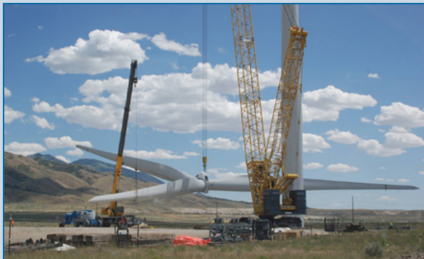
Tooele Army Depot’s second wind turbine stands 262 feet high and each blade is 165 feet long. When fully operational, the new turbine will generate 4.7 million kwh per year — enough to power 500 to 550 homes. (Courtesy photos)
