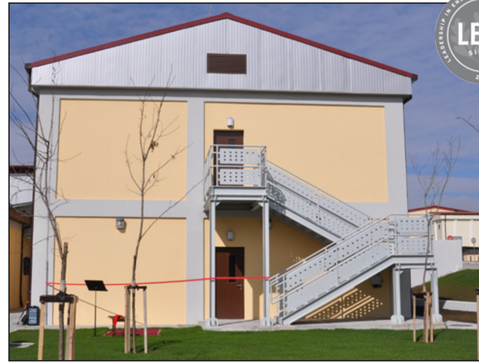
The recently completed Ankara Administrative Facility, a $1.3 million, 15,700-square-foot building, houses the legal, traffic management and post offices serving Incirlik Air Base personnel and their family members. The building officially opened March 26 and is the first LEED-certified U.S. government facility in Turkey. (Photo courtesy 39th Wing Public Affairs)
