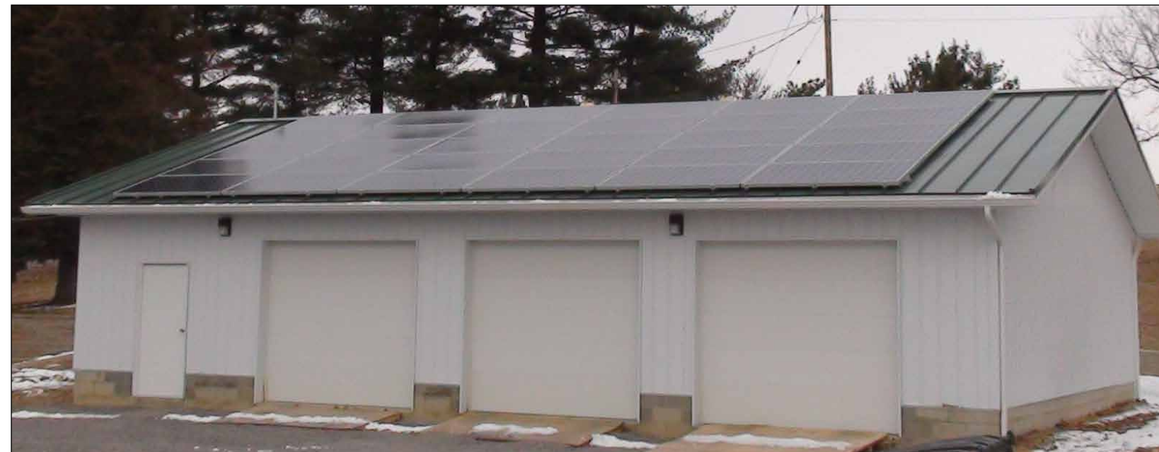
Photovoltaic solar panels installed on the roof of the maintenance shed at Beach City Lake in Beach City, Ohio. (Courtesy photo)
