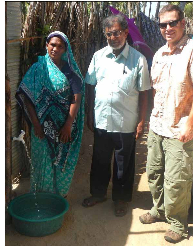
Mike MacMillan, project manager in the Environmental Special Projects Branch, poses with a newly installed water spigot near Puttalam, Sri Lanka. (Courtesy photo)
