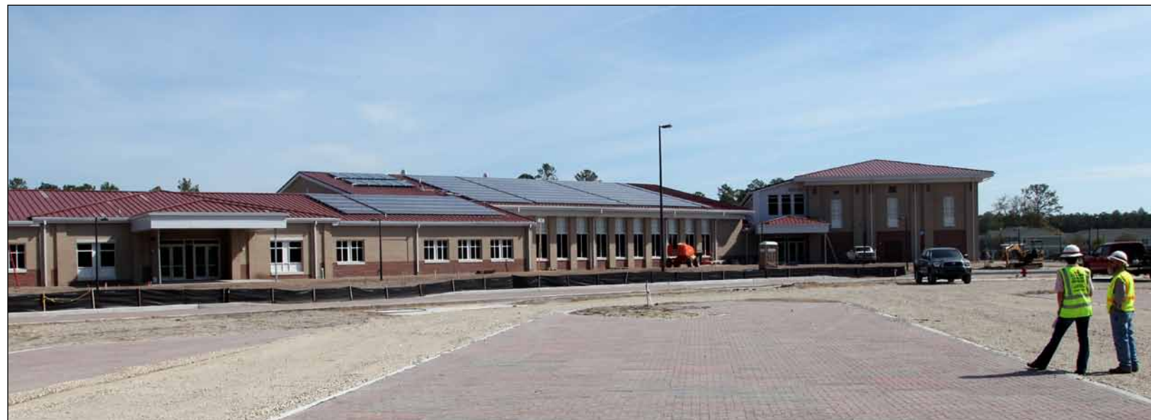
The new Murray Elementary School at Fort Stewart, Georgia, shown here in mid-April shortly before completion, includes 456 solar photovoltaic panels and 10 solar water heating panels on the roof. These panels will augment the facility’s total electrical usage and heat about 40 percent of the building’s hot water. (Photo by George Jumara)
