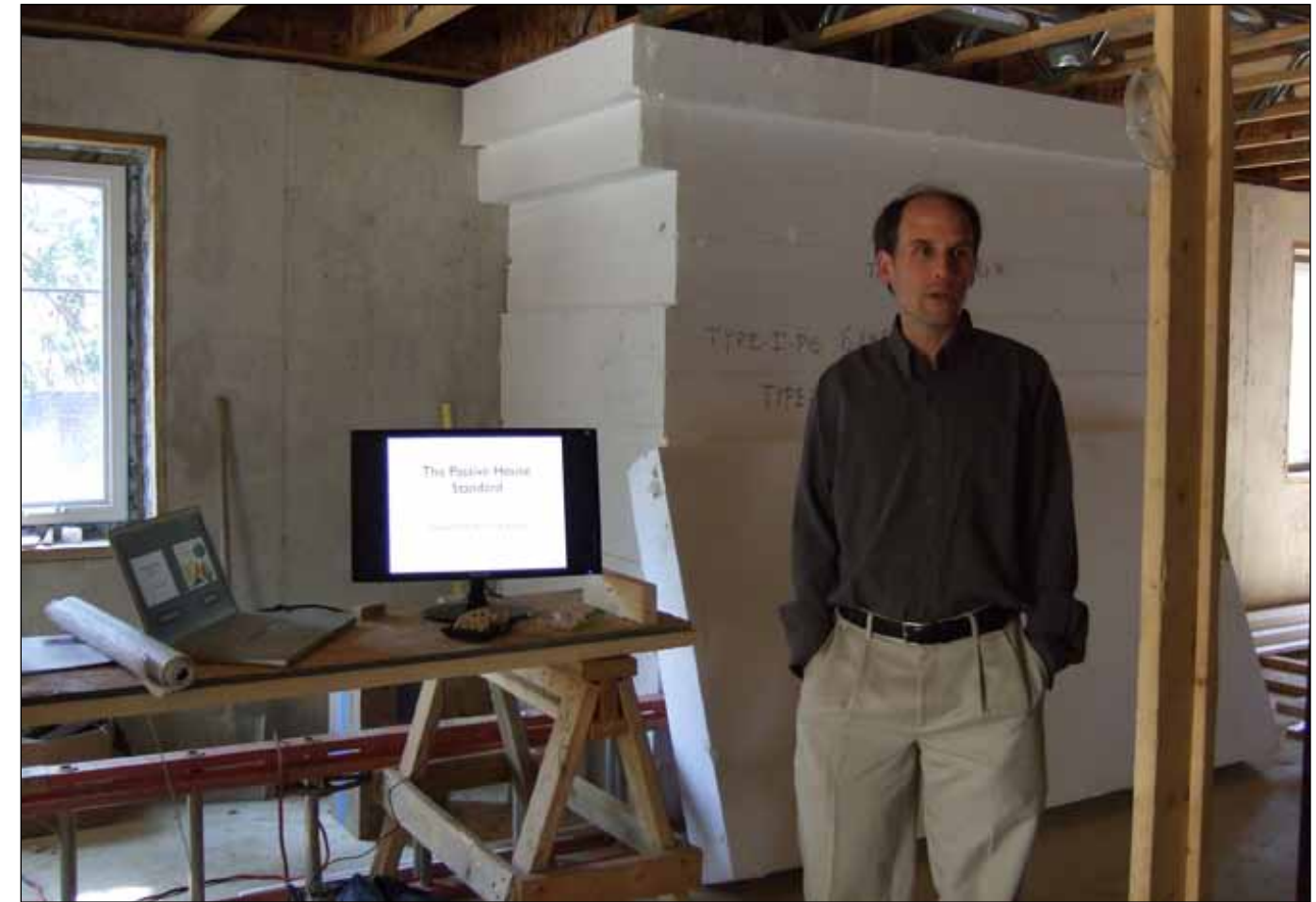
Architect Peter Henry explains PassivHaus concepts at the Labbe’s worksite. The stacks of thick foam insulation are one of the home’s key features. (Photo by Lara Beasley.)
