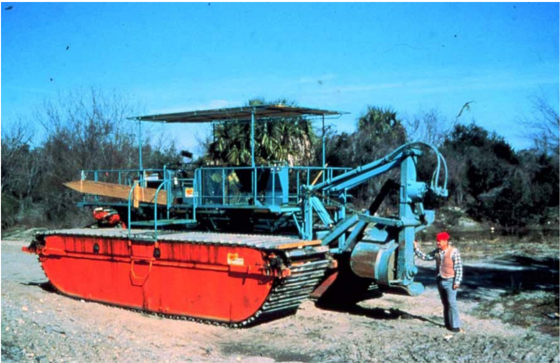
Figure 12. Track-mounted rotary trencher
