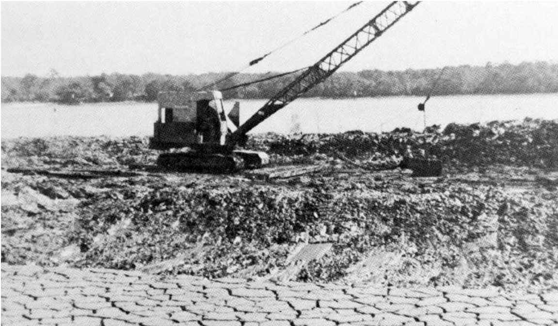
Figure 10. Small dragline operation for perimeter trenching
