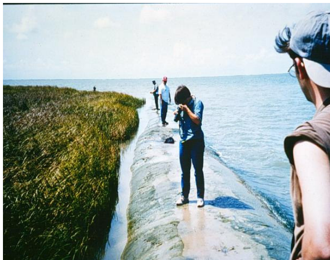
Figure 22. Salt Marsh Behind Geotube
