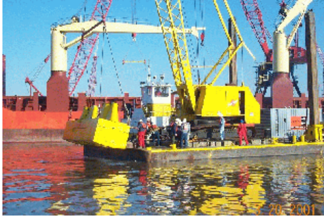
Figure 6. Deployment of the Wing Xcavator in Green Bayou, Texas
