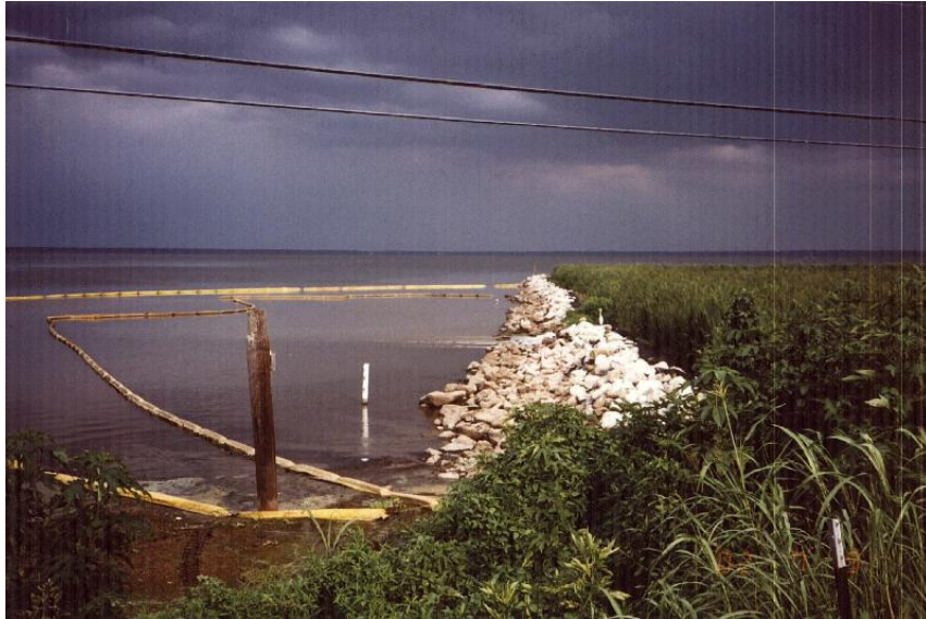
Figure 16. Silt Curtains Deployed at Lake Palourde Fill Site
