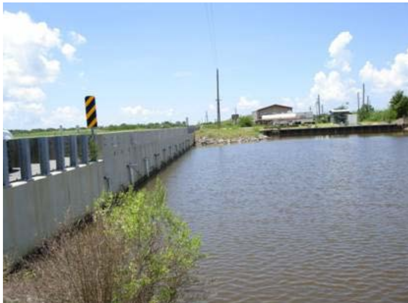
Downstream (western) side of existing Black Bayou Culvert Structure
