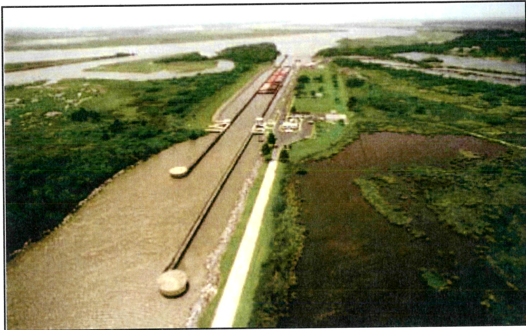
Calcasieu Lock Looking Northwest Toward Choupique Island and the Calcasieu River
