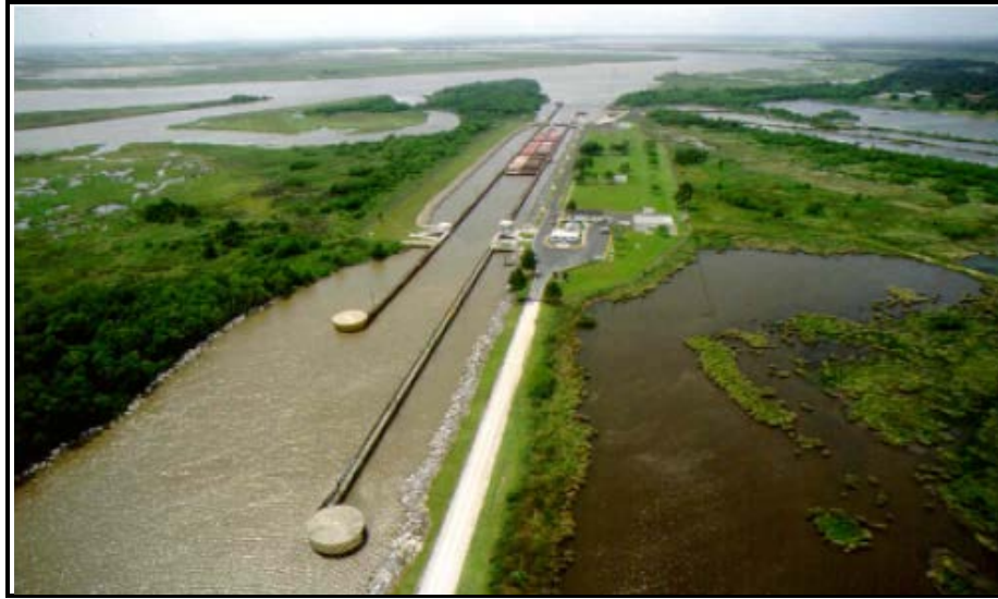
Photograph D-1. Aerial View of Calcasieu Lock
