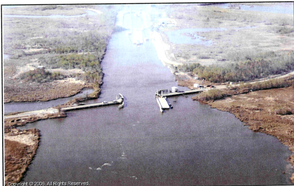
Calcasieu Lock and Pontoon Bridge Looking Southeast
