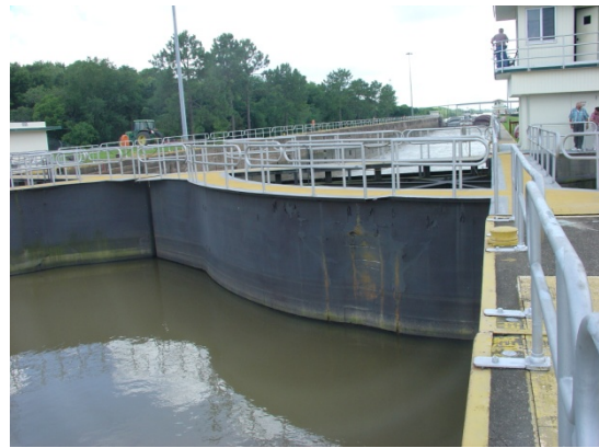
Figure 6: Top and back of sector gate, Algiers Lock Figure 7: Front of sector gate, Algiers Lock
