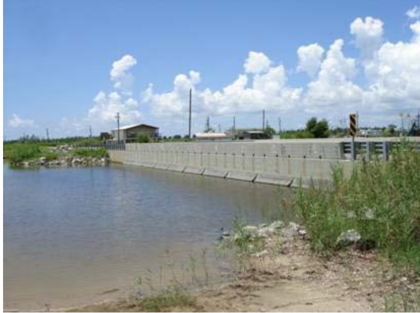
Upstream (eastern) side of existing Black Bayou Culvert Structure
