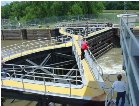
Figure 6: Top and back of sector gate, Algiers Lock Figure 7: Front of sector gate, Algiers Lock
