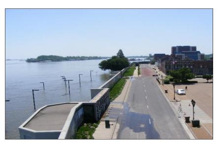
ABSTRACT: The purpose of the Project is to minimize the risk of loss of life and damages to public and private infrastructure to Paducah, Kentucky, from flooding by the Ohio River through reconstruction of an existing Corps of Engineers floodwall and levee system. The city of Paducah is the non-Federal sponsor.
