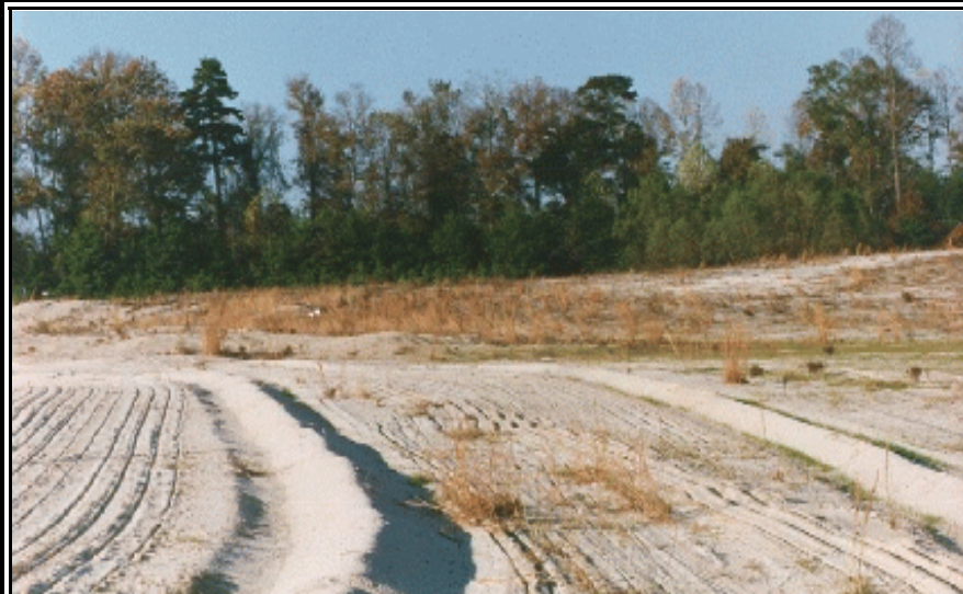
Contour Furrows - Surveyed Terrace Plow Installations
