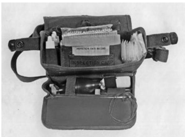
The M18 Series Chemical Agent Detector Kit was a lightweight, more sensitive, and easier use detector kit designed in 1957 to confirm the continuing presence of a chemical agent to determine when Soldiers could remove their masks.
