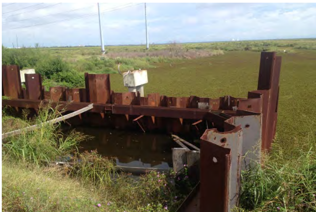
Figure 1: PS #3 Bayou Villere flood side, discharge basis covered with Salvinia sp. & Lemna sp.
