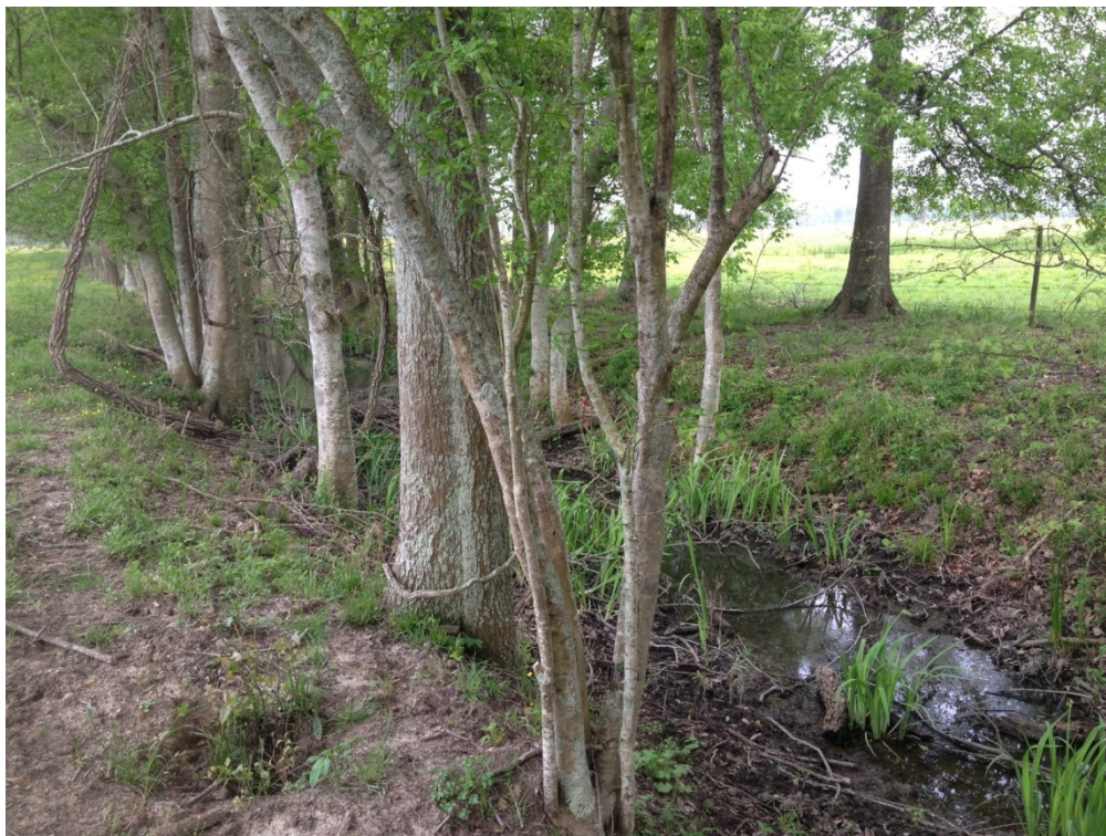
EA# 522 Mississippi River Levee, Pointe Coupee Levee July 2013
