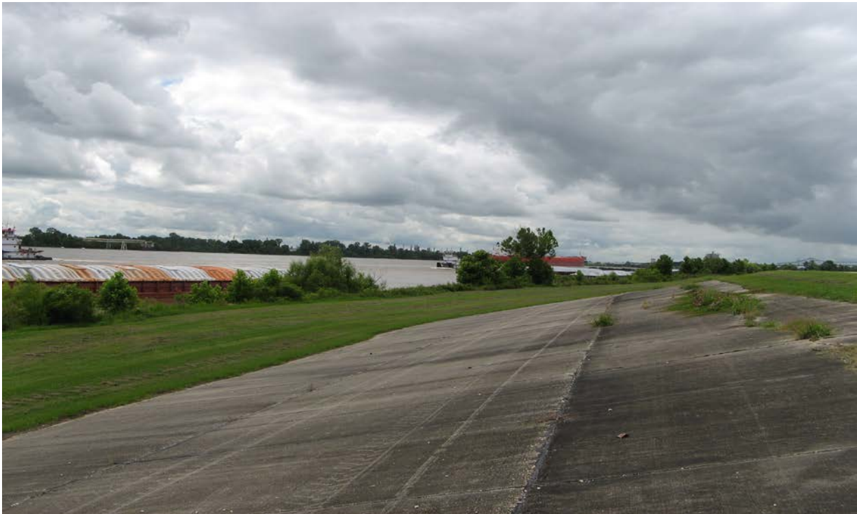
Figure 6. St. Alice stone hardpoint site existing vegetation conditions.
