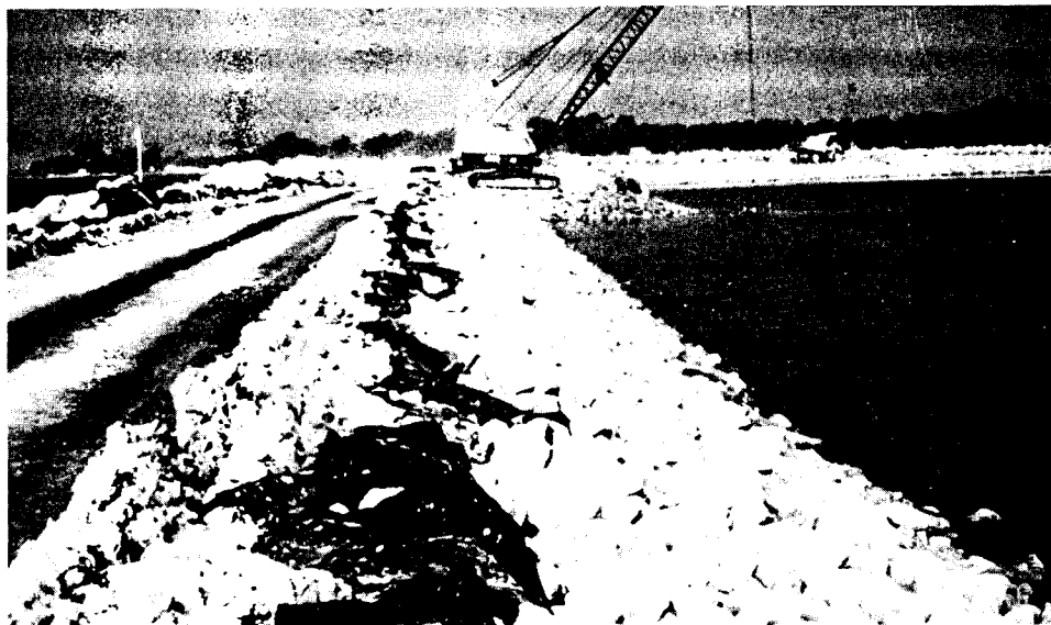
Figure 2. Dike building at Pointe Mouillee CDF in western Lake Erie. Habitat for waterbirds, waterfowl, other wildlife and fish was incorporated into the long-range management plan for the 4600-acre site
