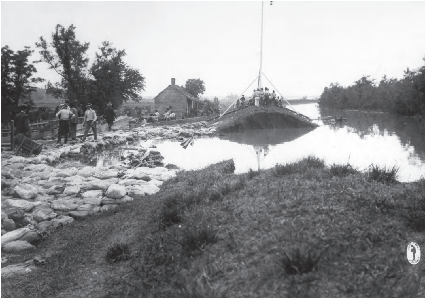
Sandbags hold back the water at a levee break at Poydras near New Orleans in May 1913.
