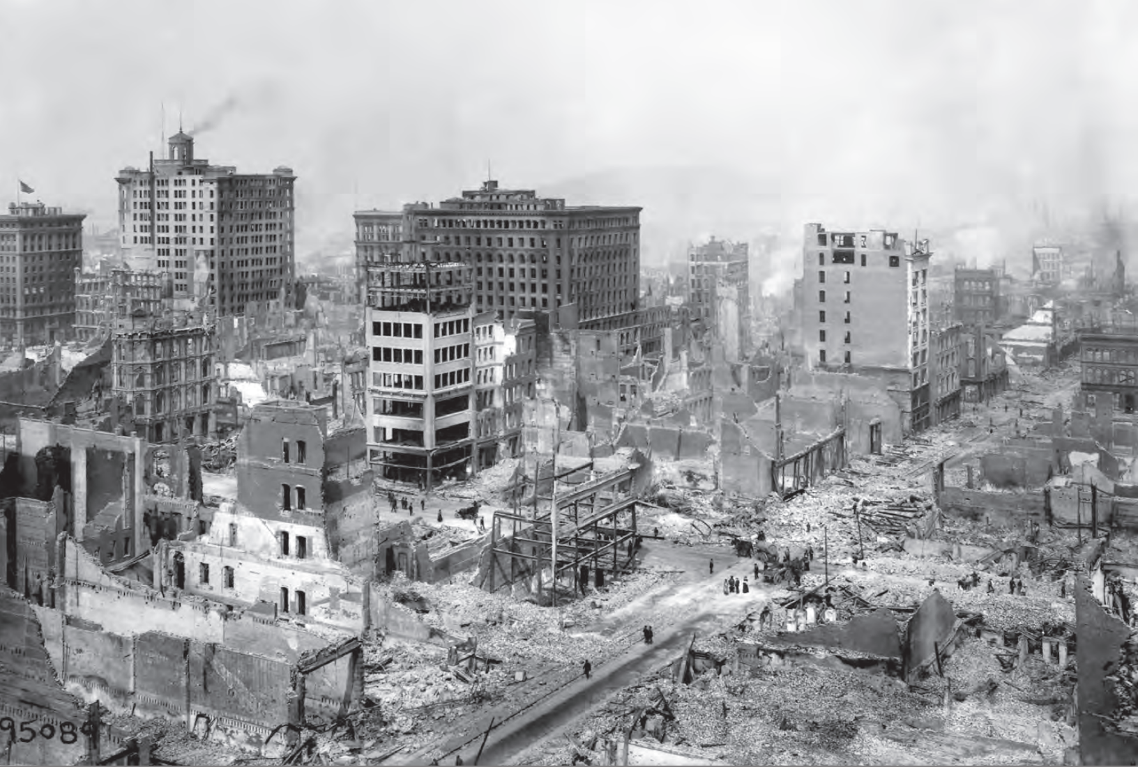
The damage to the city was extensive. Many buildings in the area north of Bush Street and east of Grant Avenue were completely destroyed.
