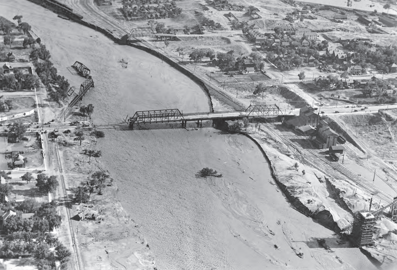
When Fountain Creek in Pueblo, Colorado, flooded in June 1921, bridges and roads were washed out.
