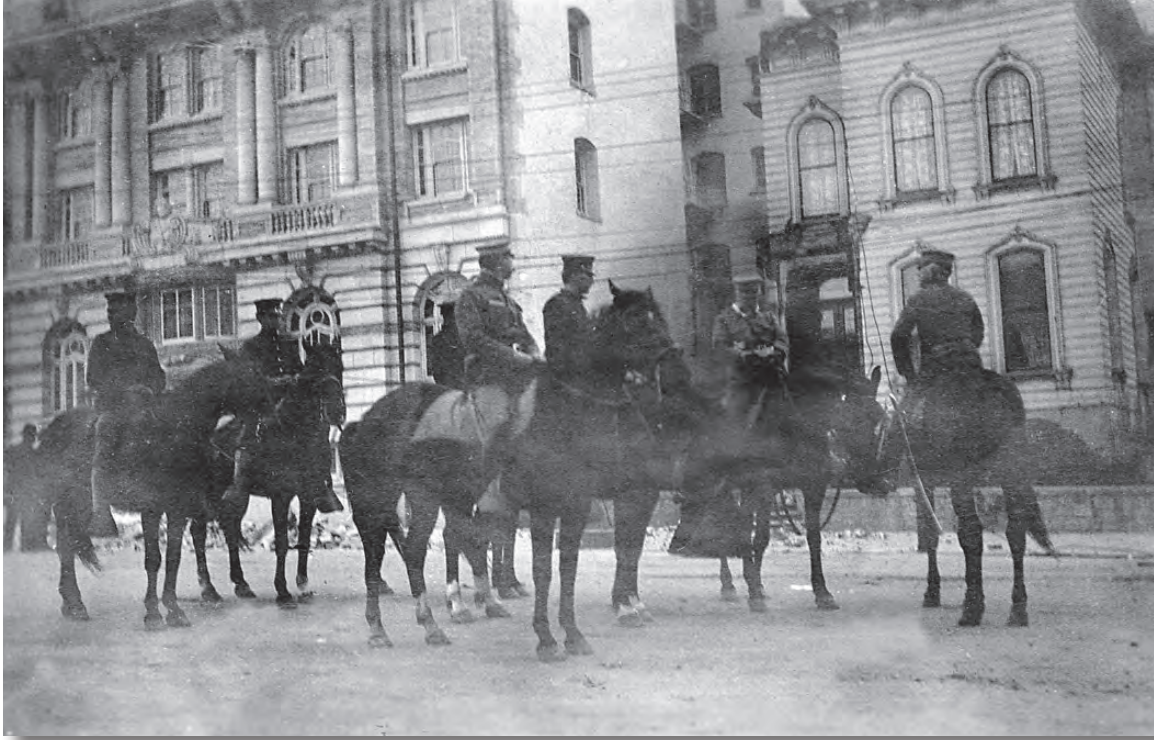
Army officers were in charge of dynamiting on Van Ness Street in San Francisco, 1906.
