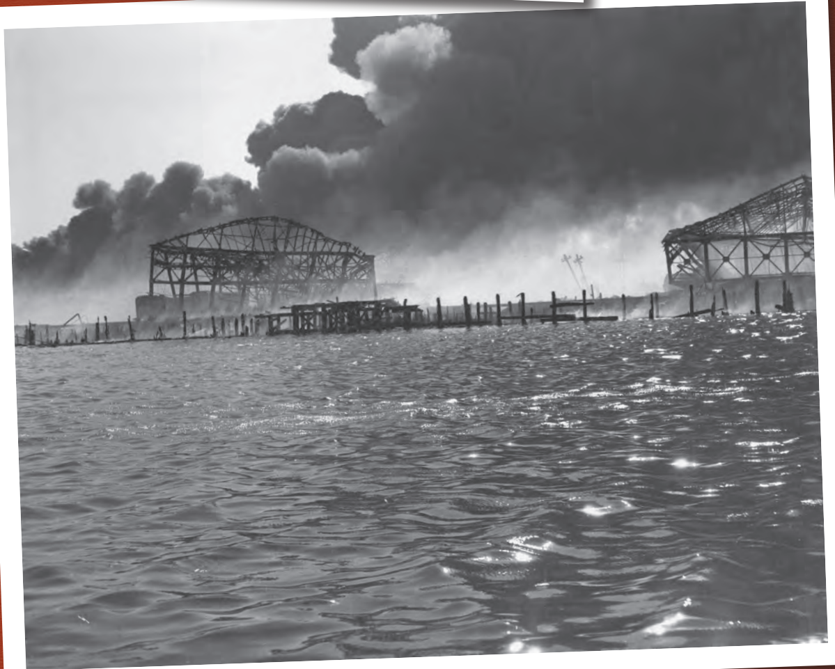
Many buildings were destroyed by the Texas City explosion, 16 April 1947.
