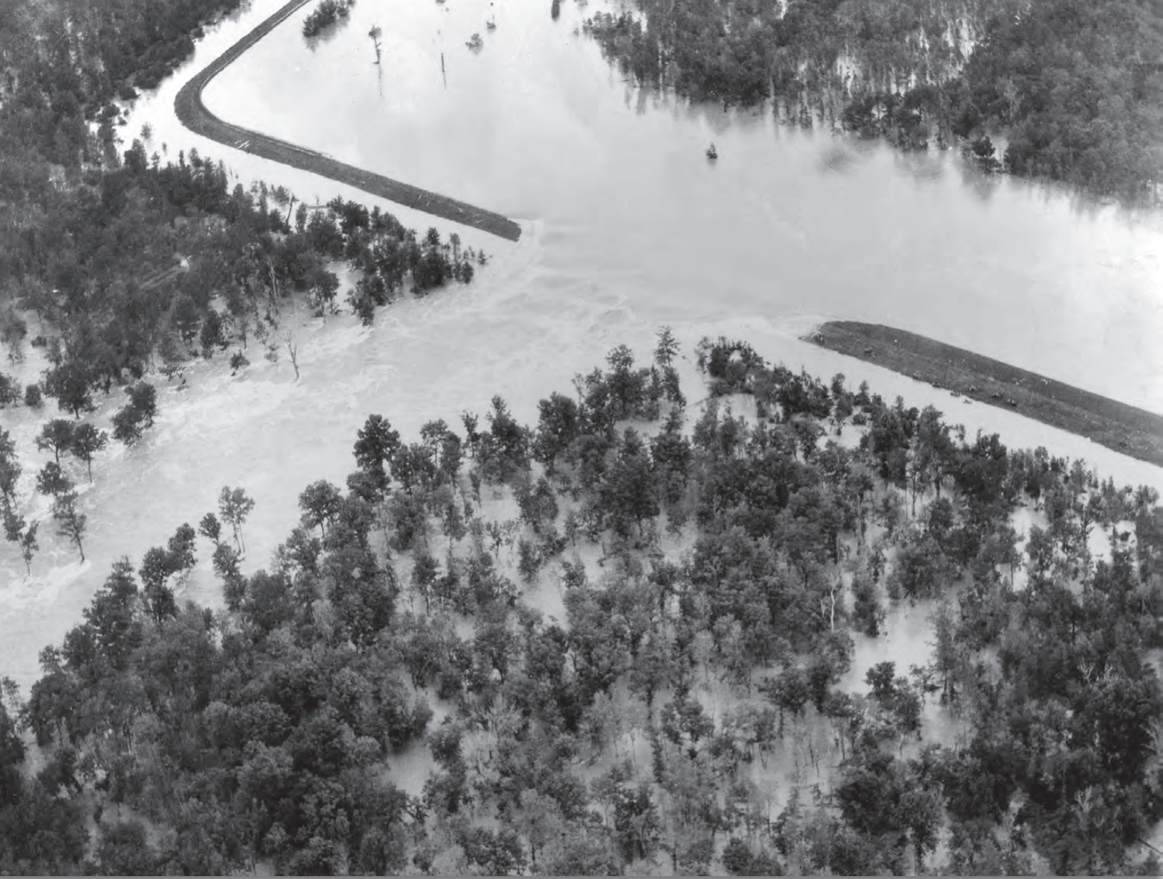
The Cabin Teele levee crevassed at Madison Parish, Louisiana, in May 1927.
