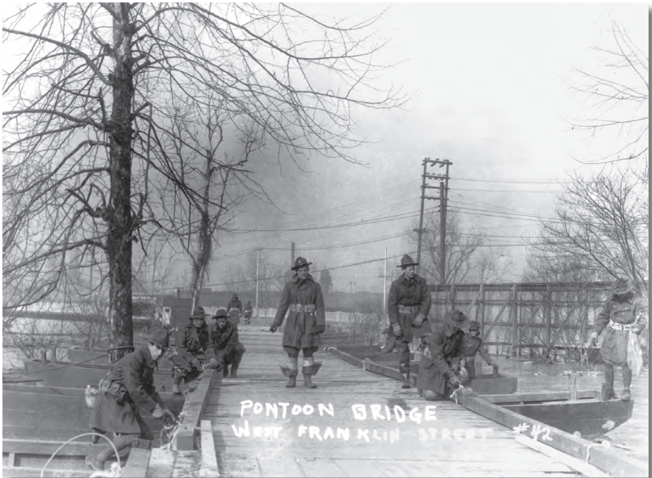
The 113th Engineers constructed a pontoon bridge in Evansville, Indiana, in 1937.
