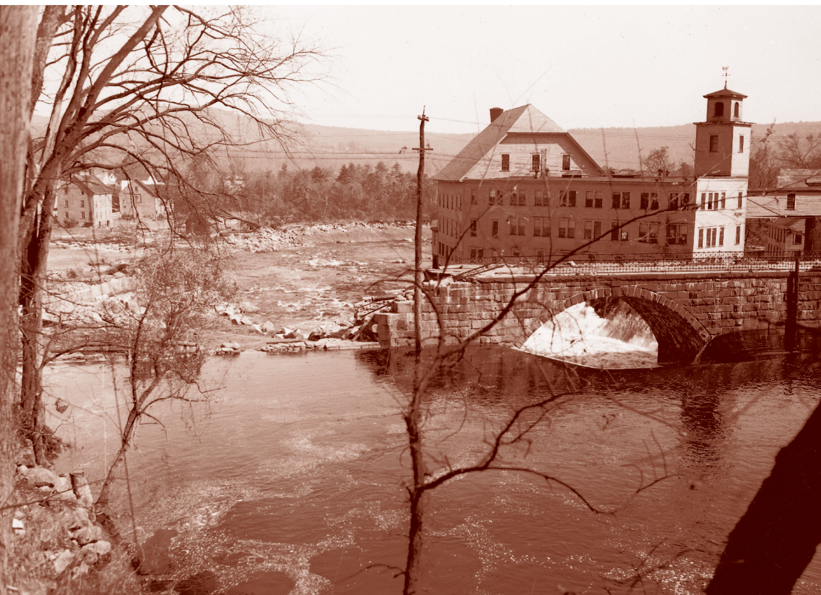
A stone bridge in Hillsboro, New Hampshire, was swept away by flooding and wind from the September 1938 New England hurricane.
