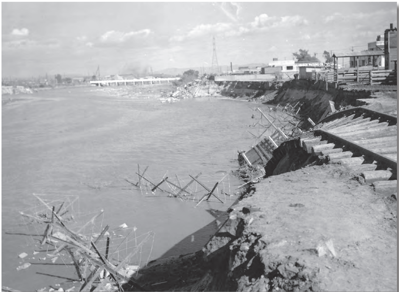
A temporary dumped-rock levee failed, causing flooding and erosion in downtown Los Angeles during the 1938 flood.
