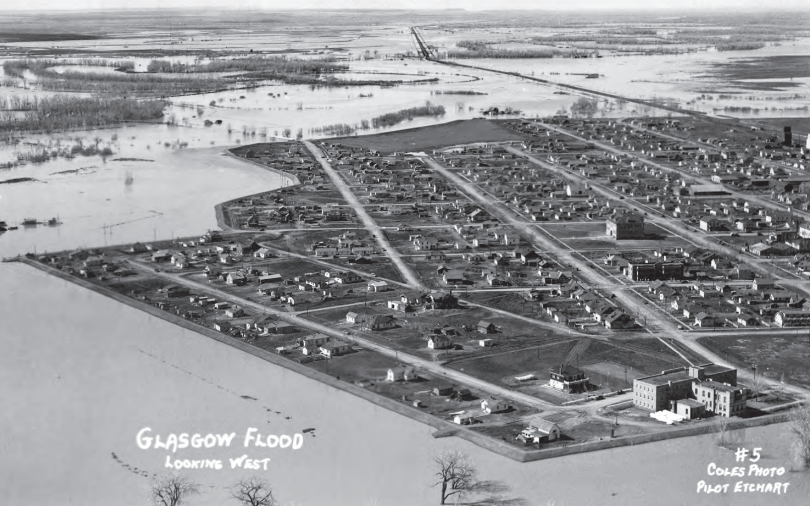
In 1939 the Corps of Engineers reinforced the levees protecting Glasgow, Montana, from flooding caused by ice dams and snowmelt. The city was nearly surrounded by water but remained dry.
