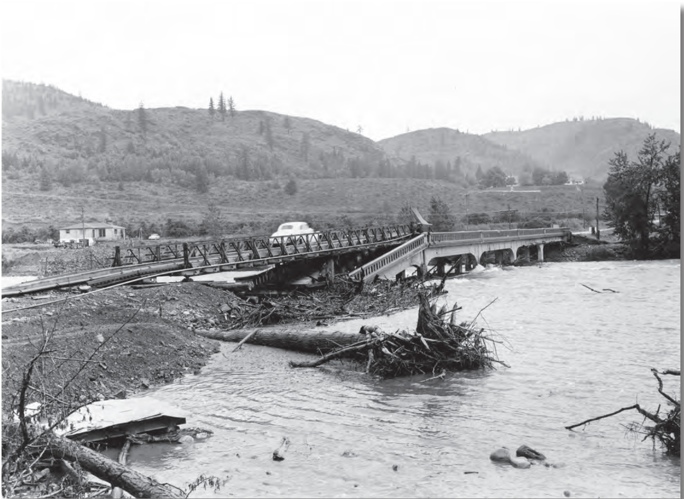
An Army Bailey bridge temporarily replaced a washed-out span over the Methow River in Washington, June 1948.
