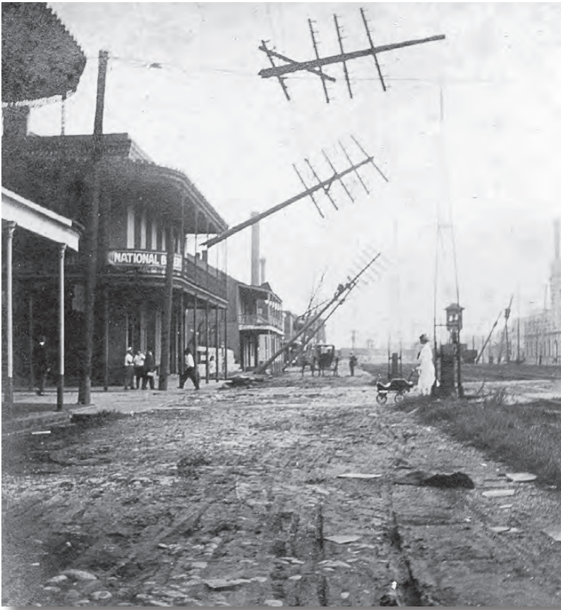
Broken utility lines dangled precariously in New Orleans, 1915.
