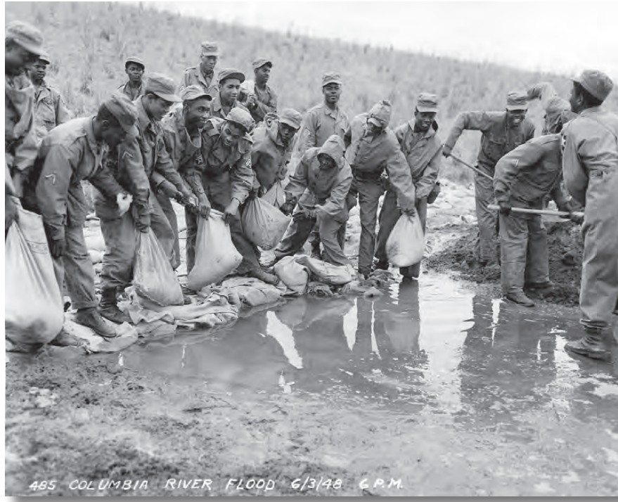
Troops of the 2d Infantry Division placed sandbags to reinforce the levee protecting Portland Air Base, threatened when the Columbia River flooded in June 1948.
