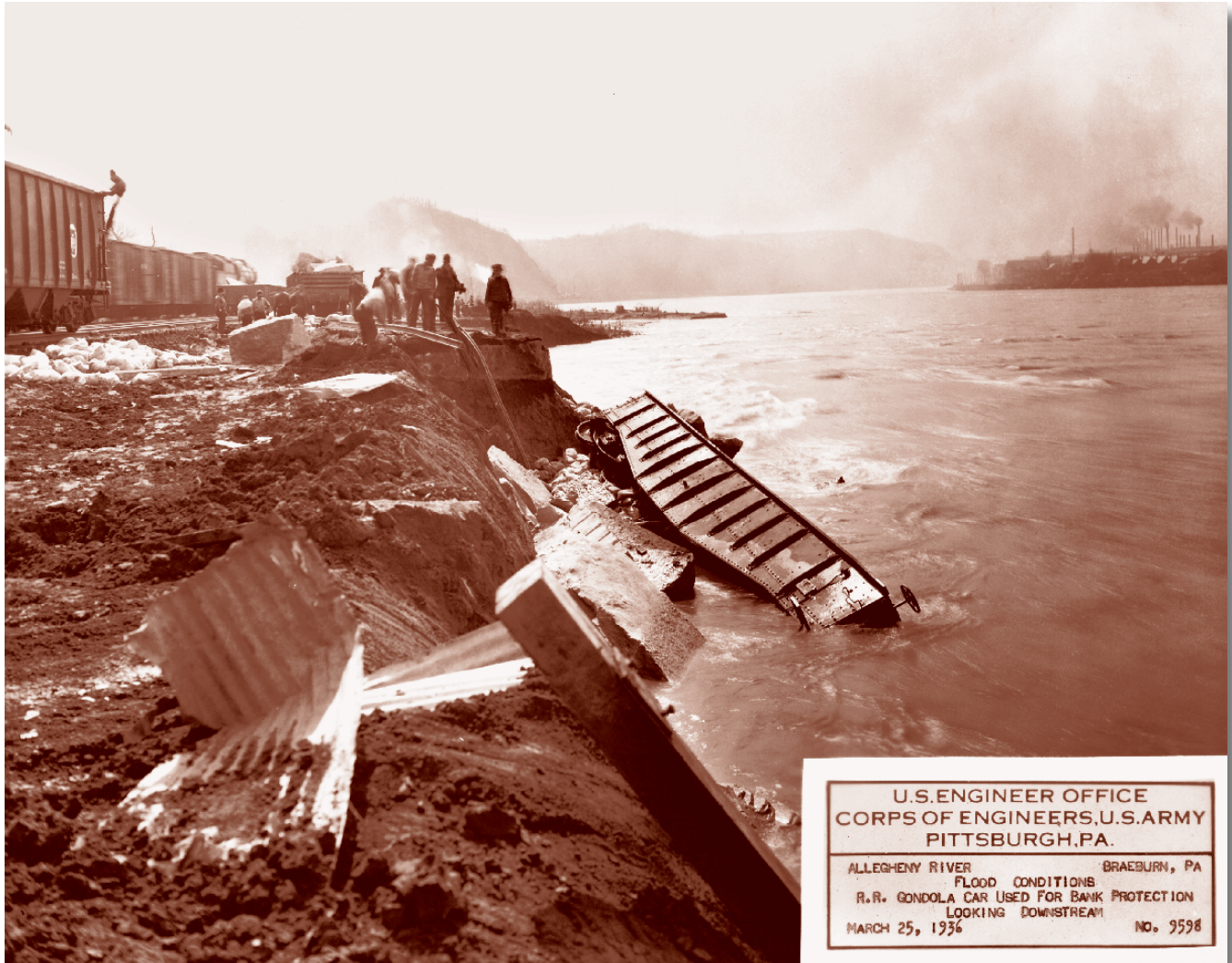
Railroad gondola cars were used for bank protection along the Allegheny River in Braeburn, Pennsylvania, 25 March 1936.
