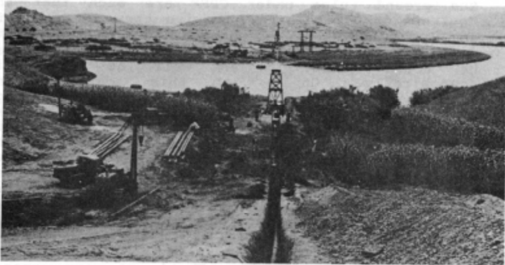
Portion of a Pipeline Linking Ben Guerir and Under Construction, 1953.
