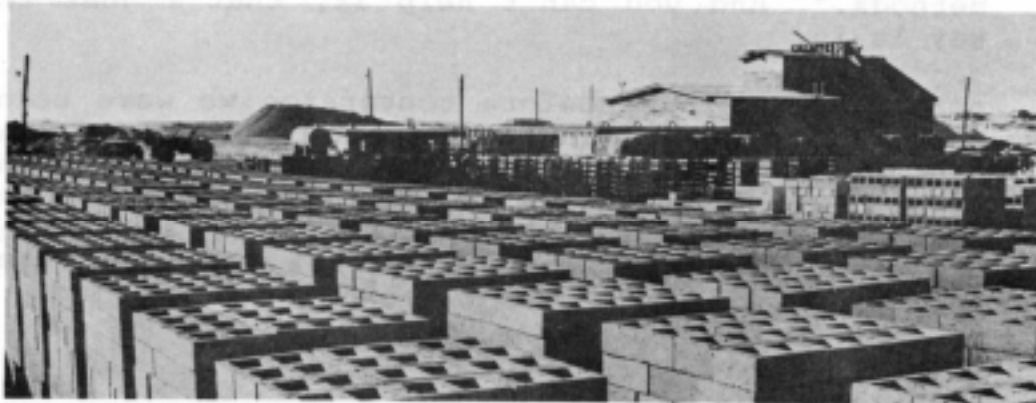
Concrete Block Plant, Dhahran Airfield, Saudi Arabia.
