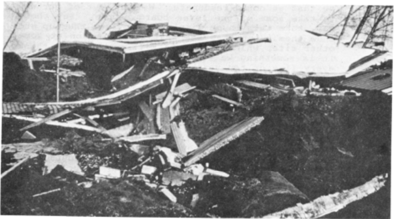
Anchorage, 1964. Residence Destroyed by Earthquake.
