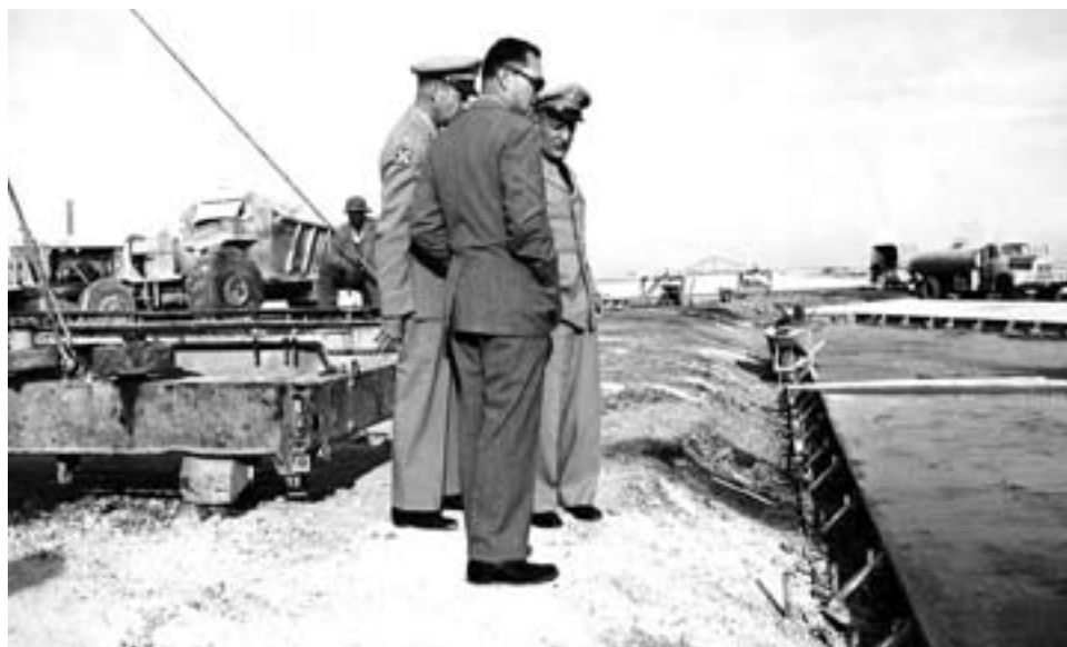
In September 1956, Chief of Engineers Maj. Gen. Emerson C. Itschner ( right ) visited Mediterranean Division headquarters at Nouasser, where he observed concrete paving of the taxiway with Lt. Col. John W. Chesley Jr., area engineer, and Paul Erskine of Atlas Constructors.
