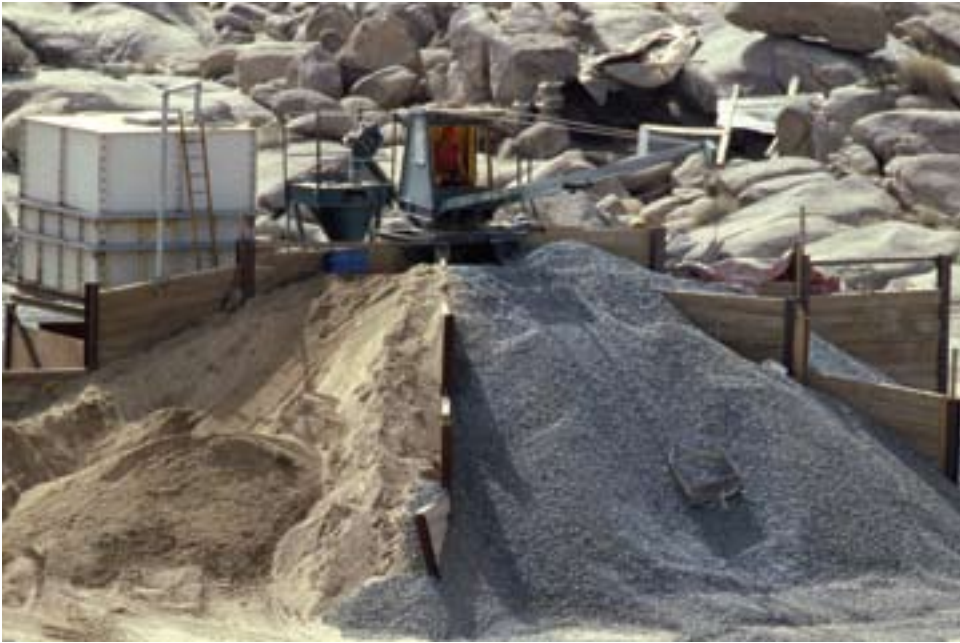
Concrete batch plant at Khamis Mushayt
