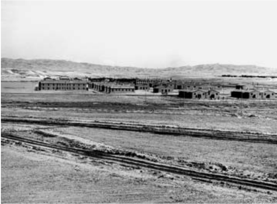
Panoramic view of the Quchan regional combat team site during construction, March 1964
