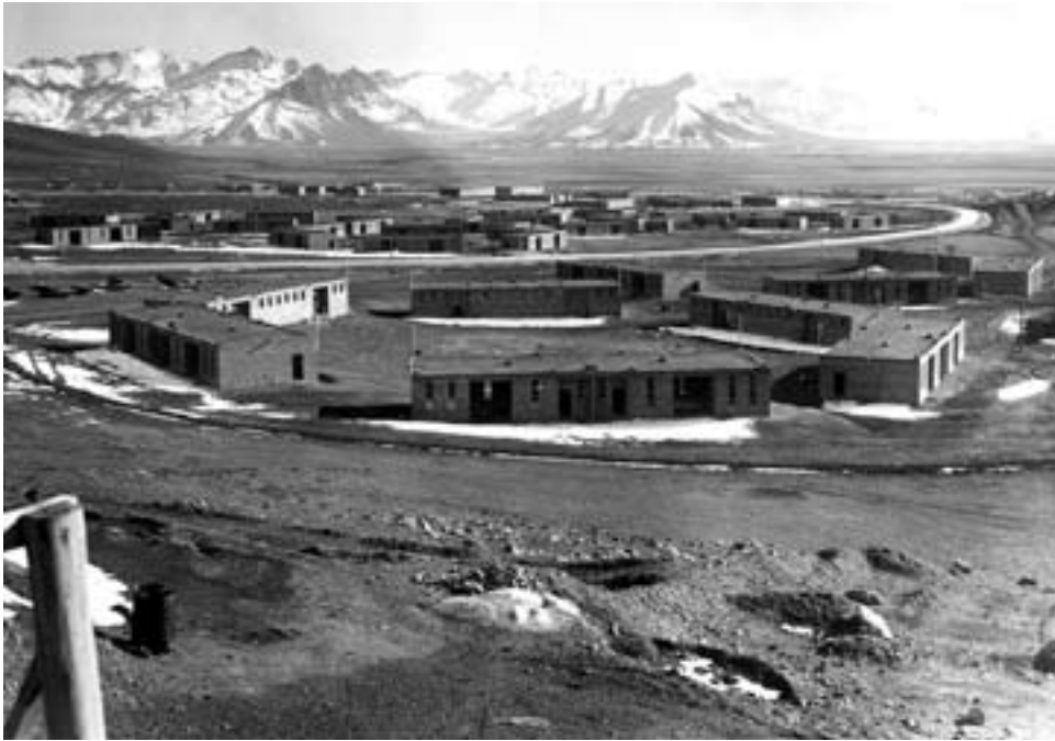
Officers quarters under construction at Naqadeh, January 1959
