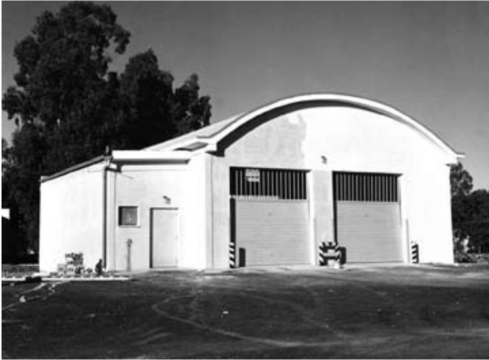
Fire station constructed under the supervision of the Brindisi field office
