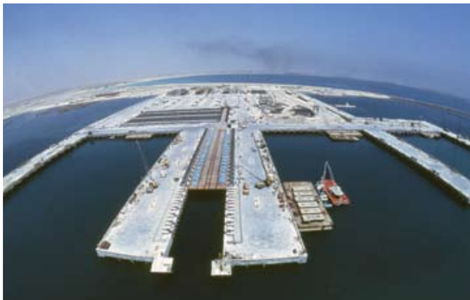
Pier piles at King Abdulaziz Naval Base, Jubayl, June 1978
