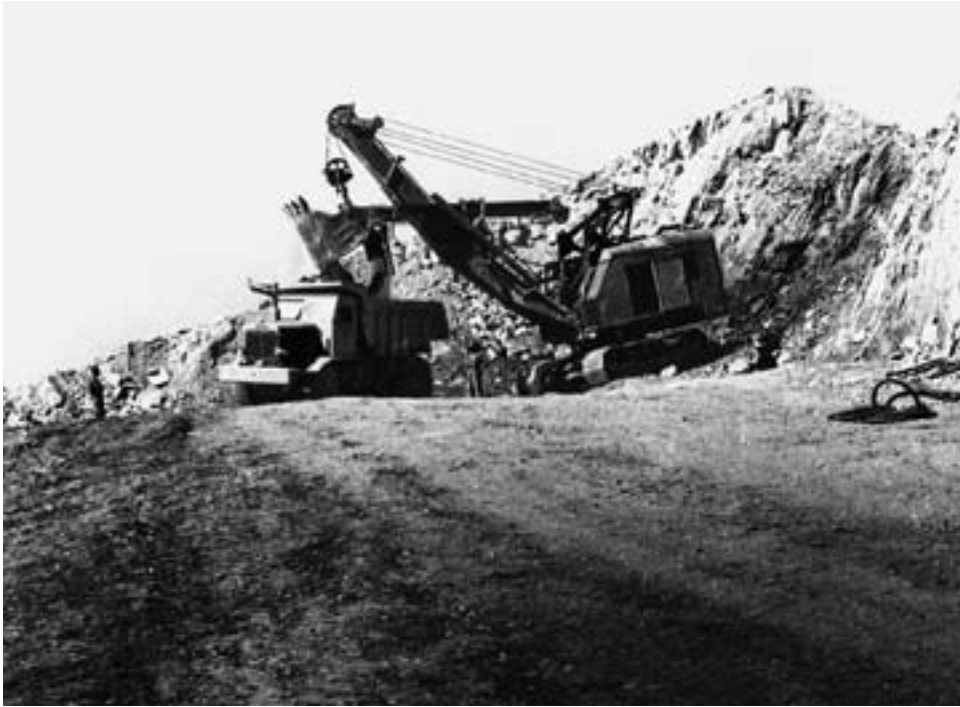
Construction of the Afghan highway, ca. 1966
