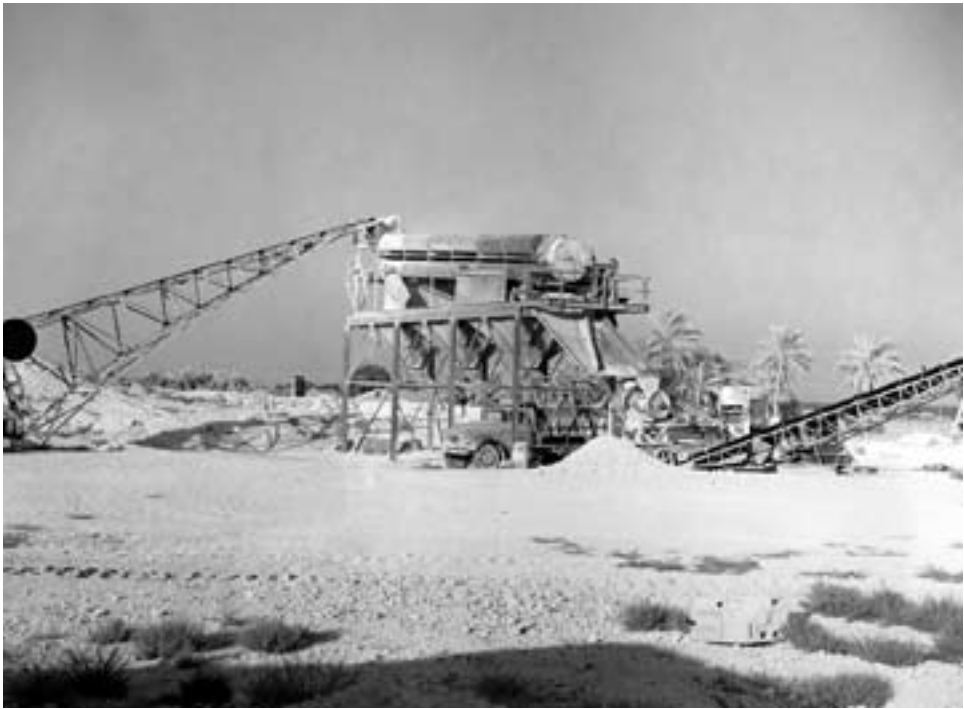
Rock-screening plant at Kharg Island
