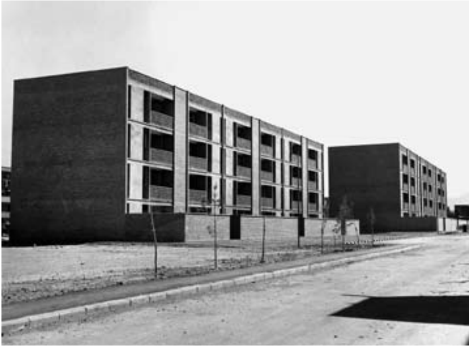
New apartment construction at Naziabad, ca. 1965
