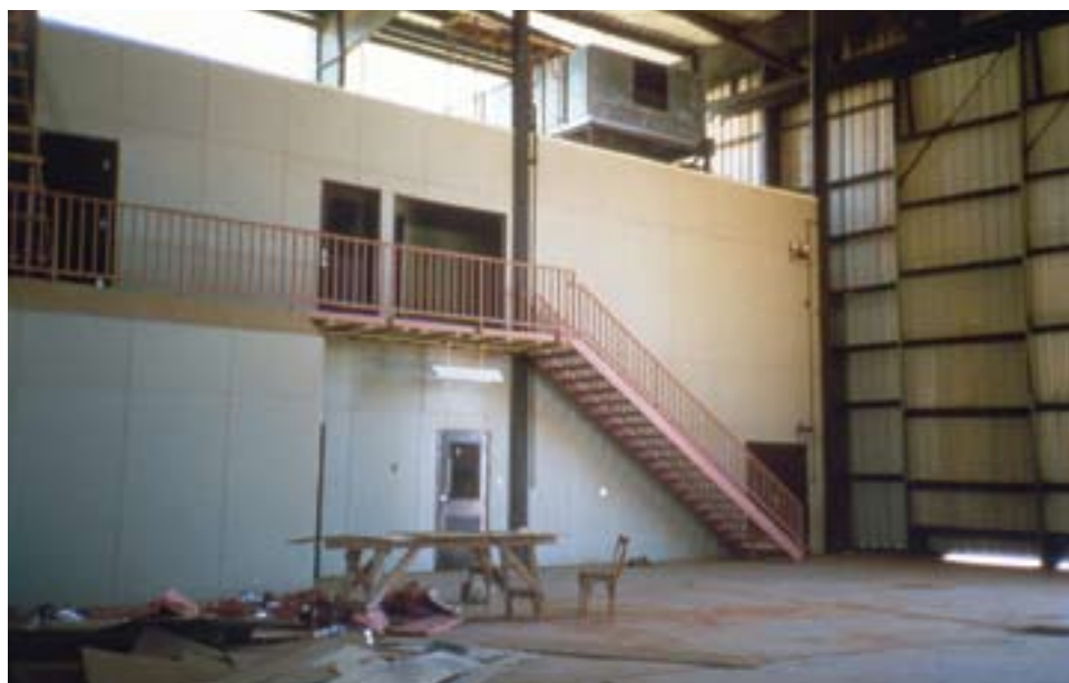
Maintenance facility near completion in Sudan, 1988
