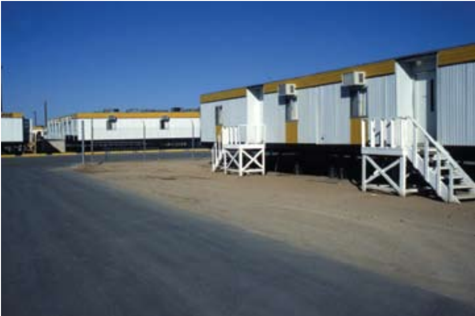
Mobilization housing at King Khalid Military City
