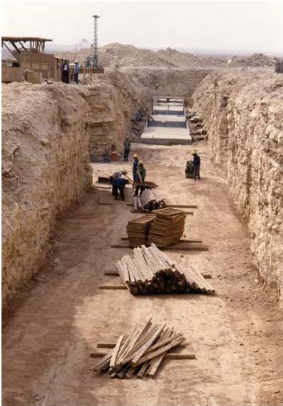
Utility trench excavation at King Abdulaziz Military Academy, early 1980s
