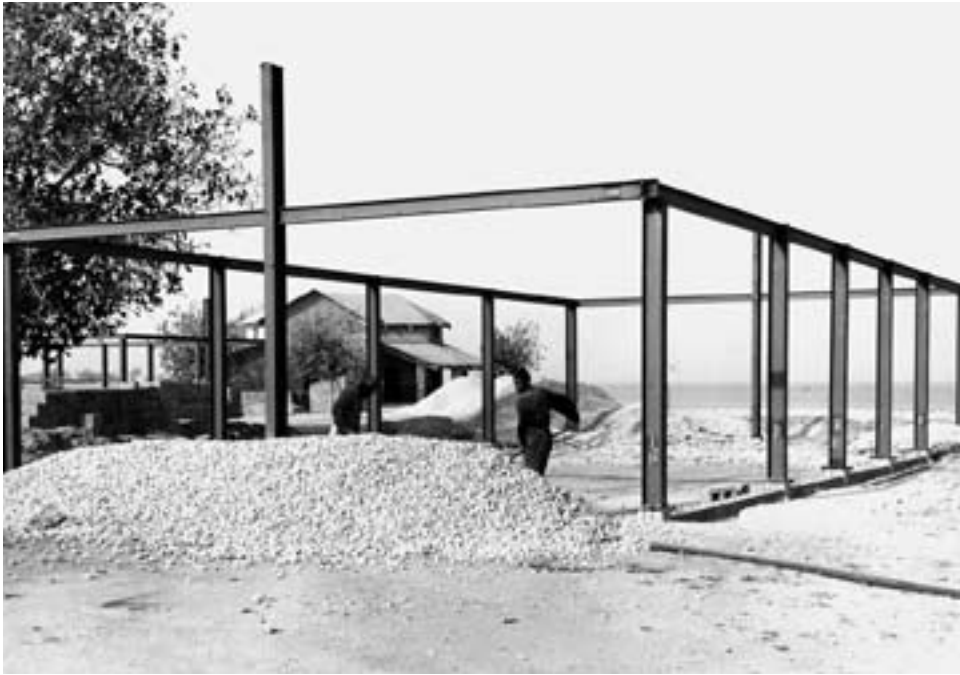
Steel framing for single-family officer quarters at Kharg Island, April 1962
