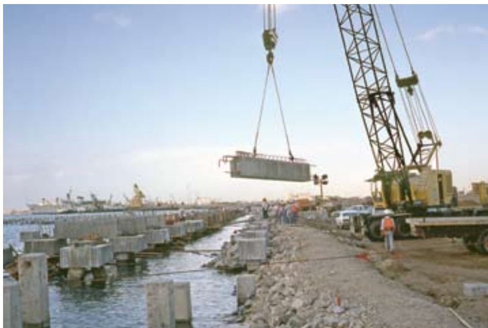
Placing a beam for the wharf at Jiddah, December 1977
