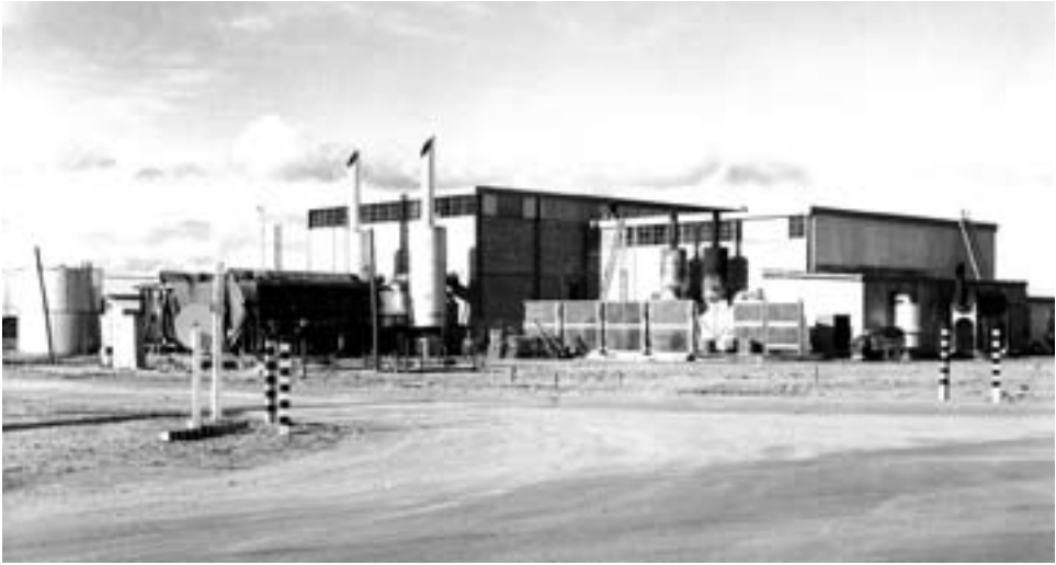
Power plant at the Sidi Slimane air base, Morocco
