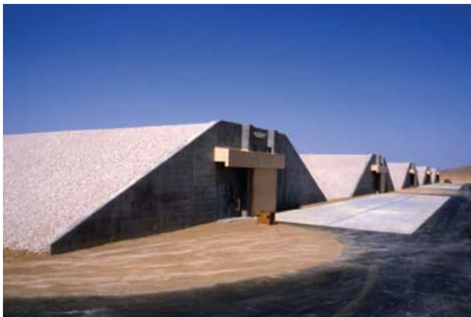
Ammo storage igloos at Thamarit
