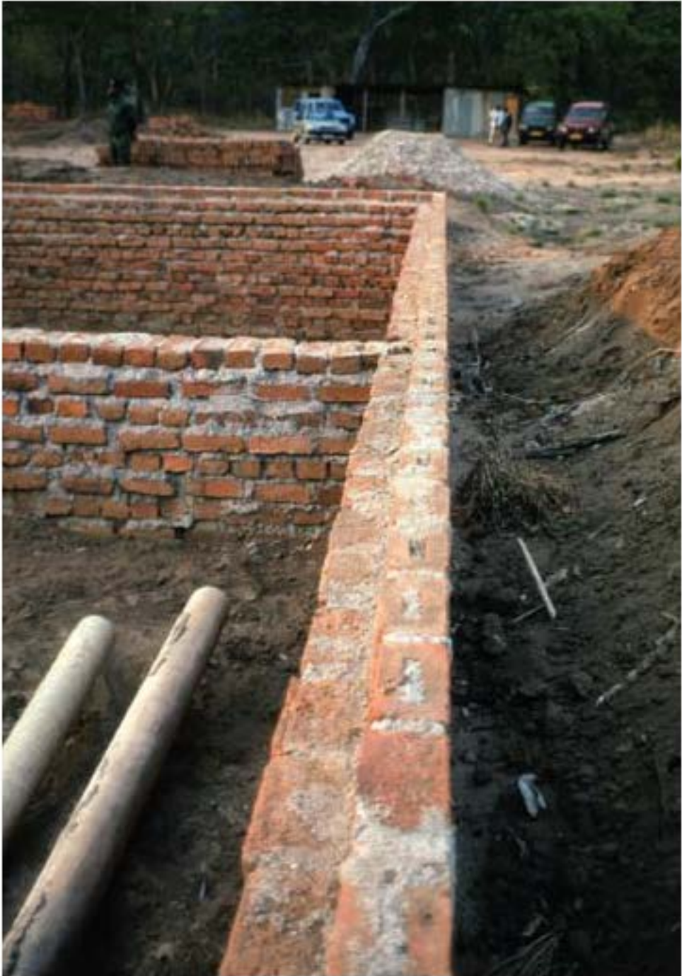
Foundation wall for medical center at Chilumba, Malawi, October 1990
