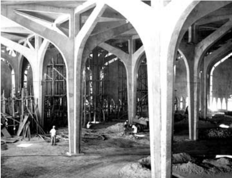
Interior of Dhahran Civil Air Terminal under construction
