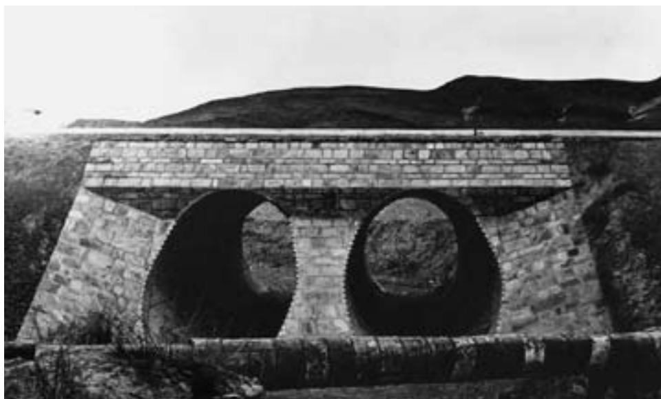
Multiplex of culverts constructed for the Afghan highway, July 1967
