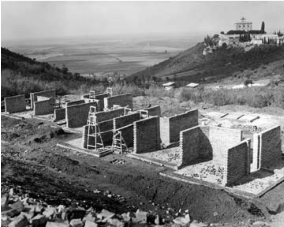
Partitions for buildings at Behshahr, Iran, were put up first while contractors waited for face bricks for the exterior walls.
