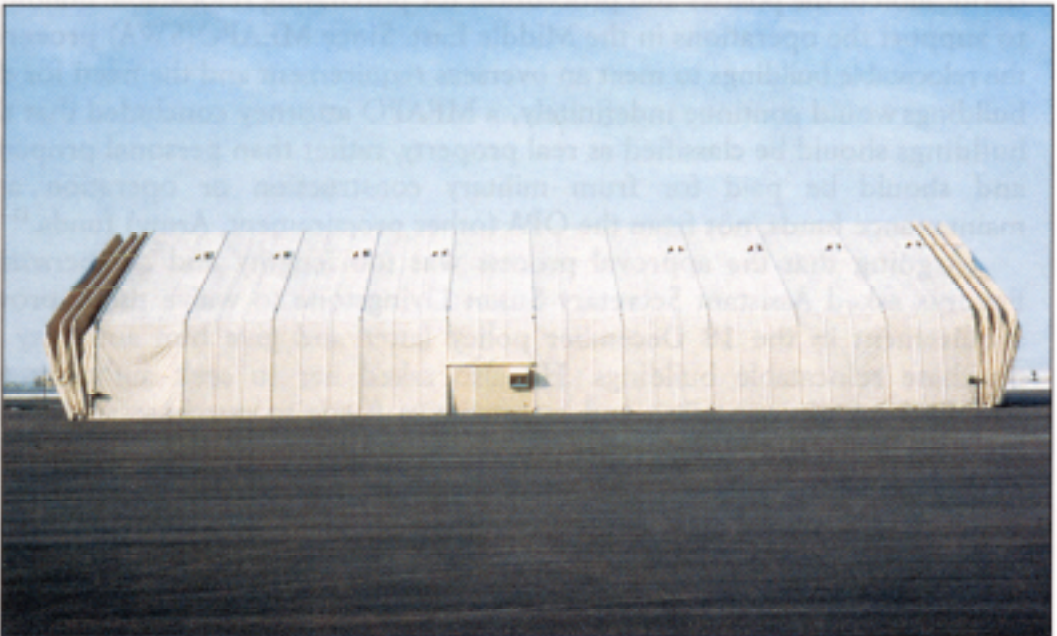
Side view of a clamshell building at King Fahd International Airport. The ends of the clamshell are opened and closed by either a band-cranked or a generator-driven winch.
