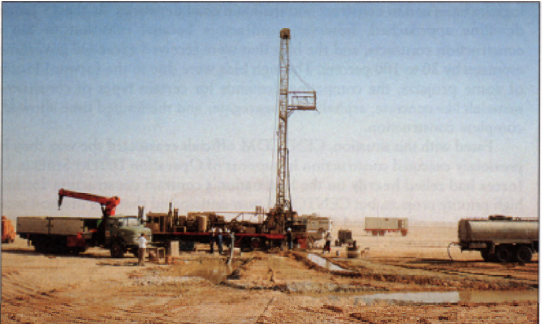
A contractor drills for water in the Saudi Arabian desert.
