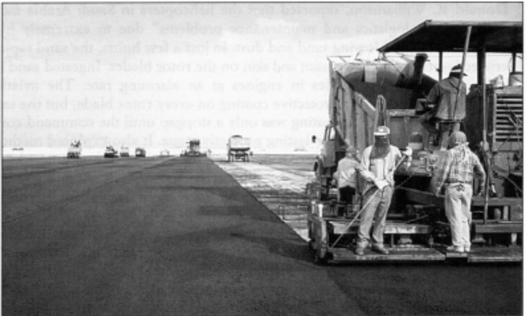
Two asphalt paving machines work side by side at the King Fahd International Airport. Five of these machines were used simultaneously to handle the daily requirement of
