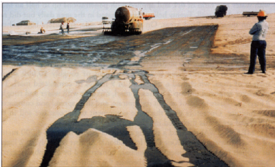
Emulsified asphalt was used as a dust palliative at Thadj.
