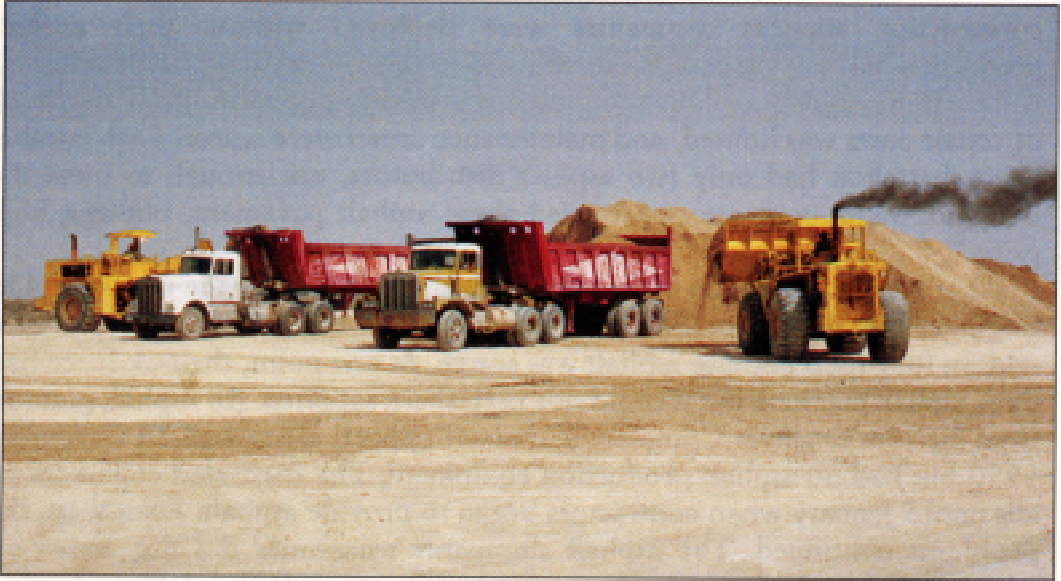
Base course stockpile area for work at KingFahd International Airport. The lack of an adequate source of base course in the eastern province of Saudi Arabia forced contractors to haul material from Abu Hadryiah, 100 kilometers away.
