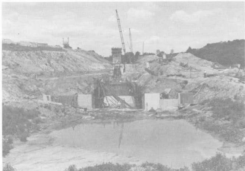
The La Farge lake and dam under construction in June 1973. The Corps stopped construction in April 1975 because of opposition from environmental groups and Wisconsin state officials.
