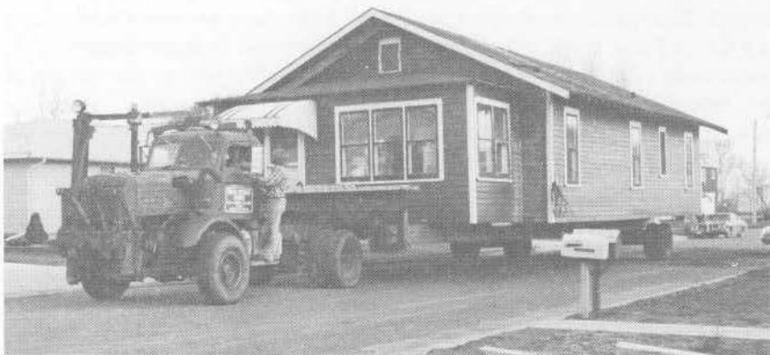
The relocation of Prairie du Chien in 1978 — a house-by-house solution to the flooding problem.
