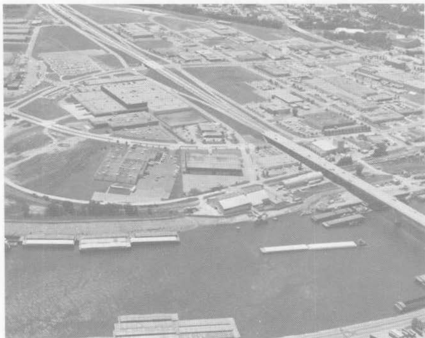
The St. Paul industrial floodplain in 1981. The "new" bridge is at far right. The levees and floodwalls are visible along the river.
