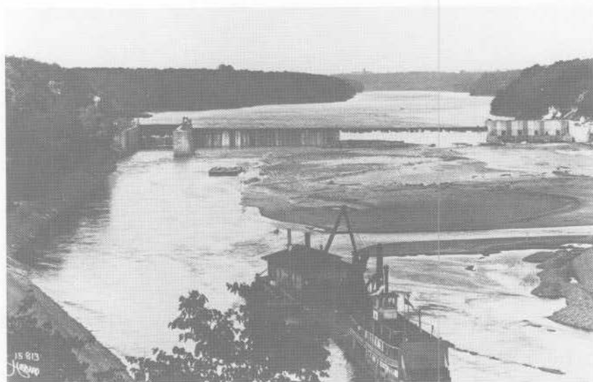
Twin City Lock and Dam No. 1, also known as Lock and Dam No. 1, the "high" dam, or the Ford dam, is located six miles below the Falls of St. Anthony. In the late 1920s, sewage and industrial wastes from both Minneapolis and St. Paul collected in the river above the dam.
