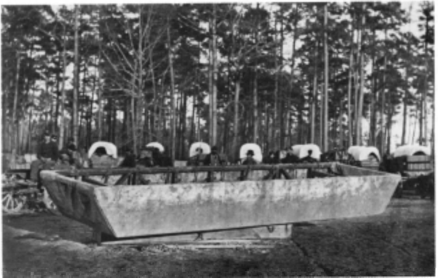
Canvas ponton, Fiftieth New York Volunteer Engineer Regiment, Rappahannock Station, Virginia, March 1864. Library of Congress photograph
