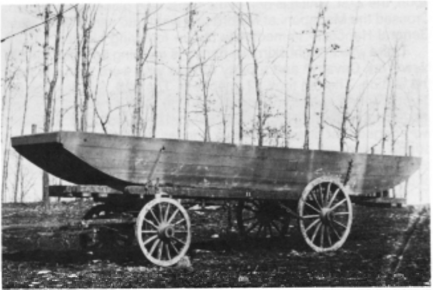
Ponton wagon and wooden ponton, Fiftieth New York Volunteer Engineer Regiment, Rappahannock Station, Virginia, March 1864. Library of Congress photograph B8184-7160.
