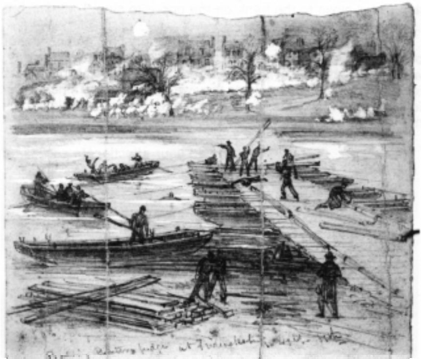
Sketch of Engineer troops laying ponton bridge at Fredericksburg, Virginia, 11 December 1862, by Alfred R. Waud. Library of Congress photograph Z62- 7023.
