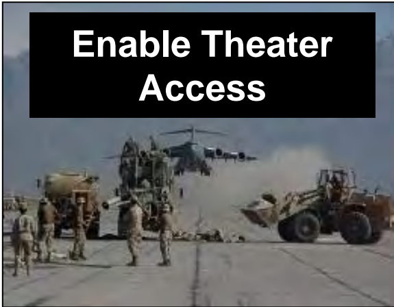
Rapid Airfield Construction
